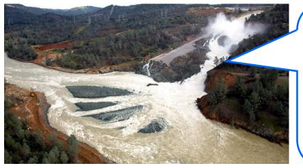
Alternative flow channel formed by erosion after failure of the spillway chute. Note the debris in the river channel, which was responsible for raising tailwater levels.
