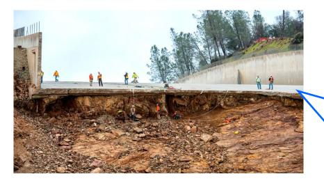
Inspection of the problem area when spillway gates were closed. Note relatively thin slab and erosion of the weathered foundation rock.
