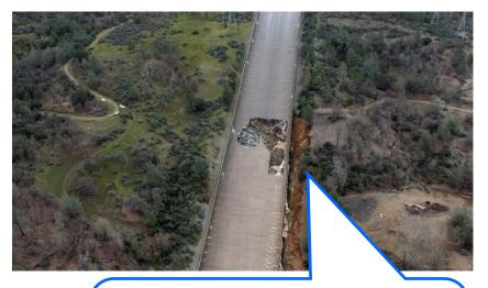
After the spillway gates were closed, the condition of the spillway was assessed. Note the missing and broken chute slabs and the erosion progressing behind the left sidewall.
