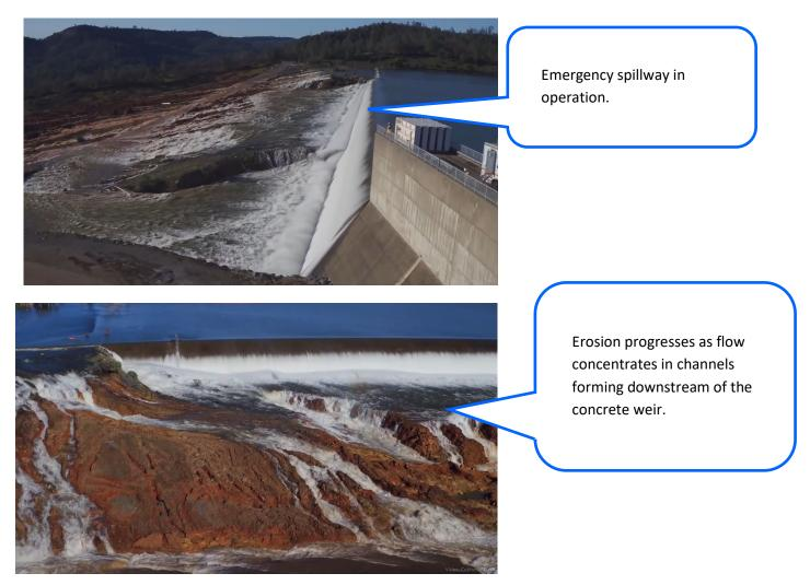
The service spillway continued operating until the flood passed and reservoir levels lowered. The erosion did not progress upstream towards the gate structure and the evacuation order was lifted two days later.
