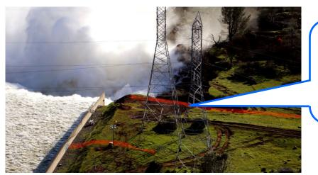
The erosion came close to the transmission towers but did not undermine the structures.
