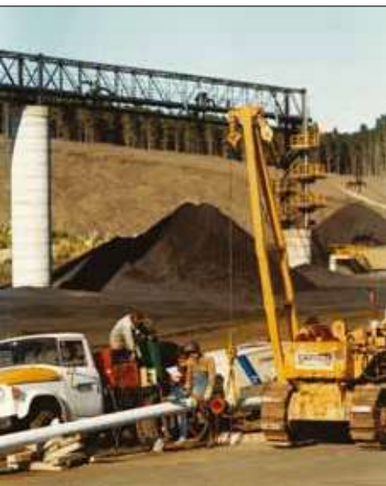
Above: Pipeline coupling being prepared by McConnell Dowell.
