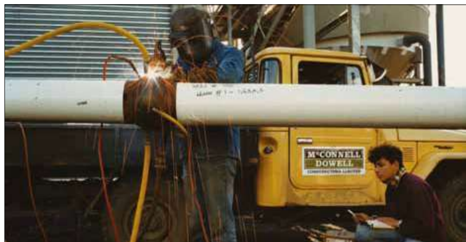
Above: Pipeline coupling being prepared by McConnell Dowell.
