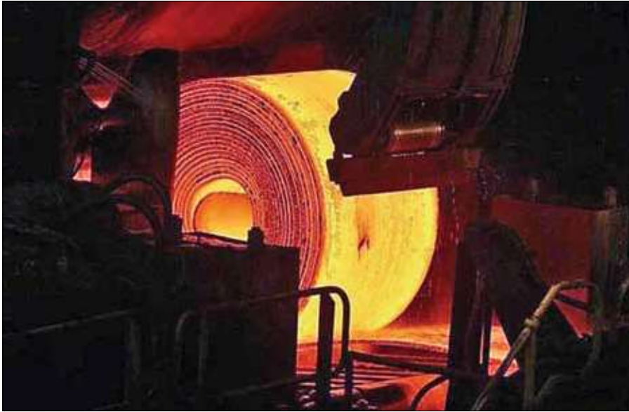
Hot Coil Box in rolling mill.
