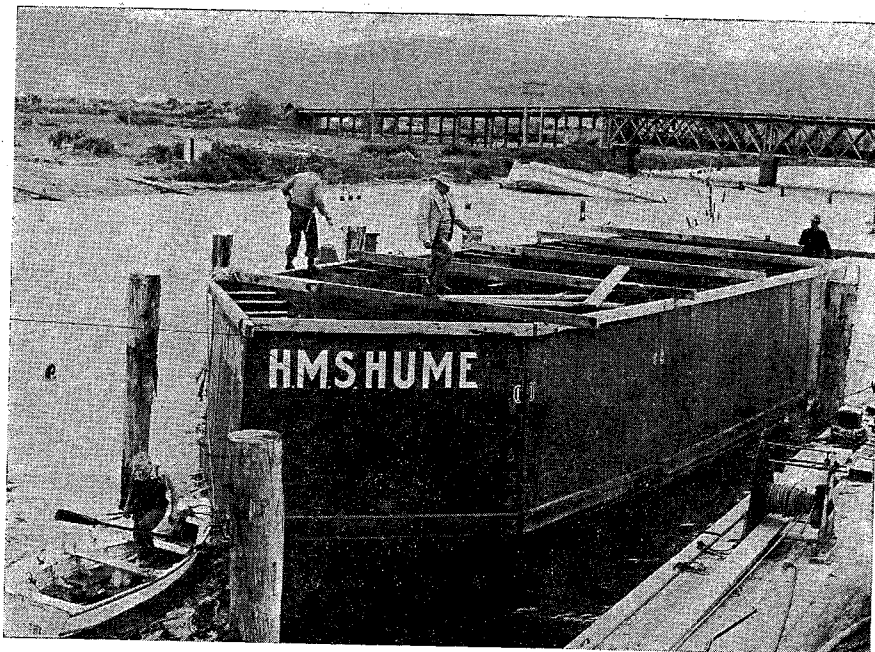
Fig. 3.—Caisson ready for sinking to position.
