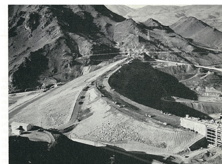
Fig. 2: Placing operations, February, 1964. (Downstream is to the right of the picture).
