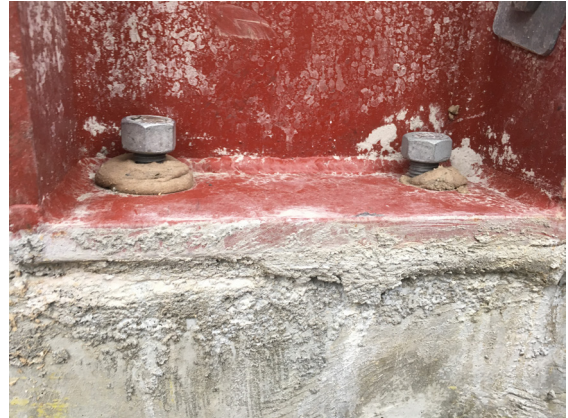
Figure 6: Portal toes to outside, nuts undone
