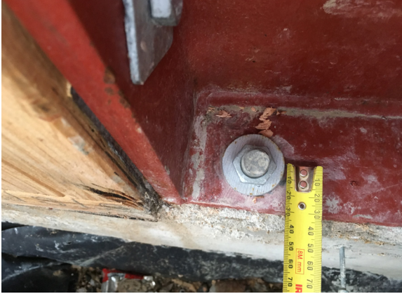
Figure 5: Portal toes to outside, insufficient edge distance
