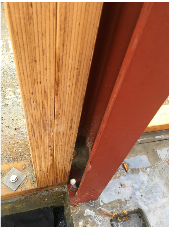
Figure 7: Portal toes to outside, edge distance, studs bent
