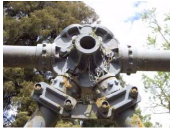
Figure 9: Detail of top chord joint on Inglis Bridge 2014
