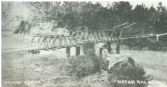
Figure 8: Rangitikei Bridge at Vinegar Hill from Scally, Hunterville & District, undated picture
