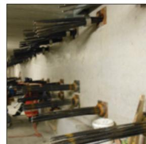
**Figure 13 –(left to right); reinforcing cage for first segment at eastern toe that eventually extended up to the hollowcore floor at the top of the picture, post-tensioned tendons ready to be cut and grouted, completed excavation of western segment.**
