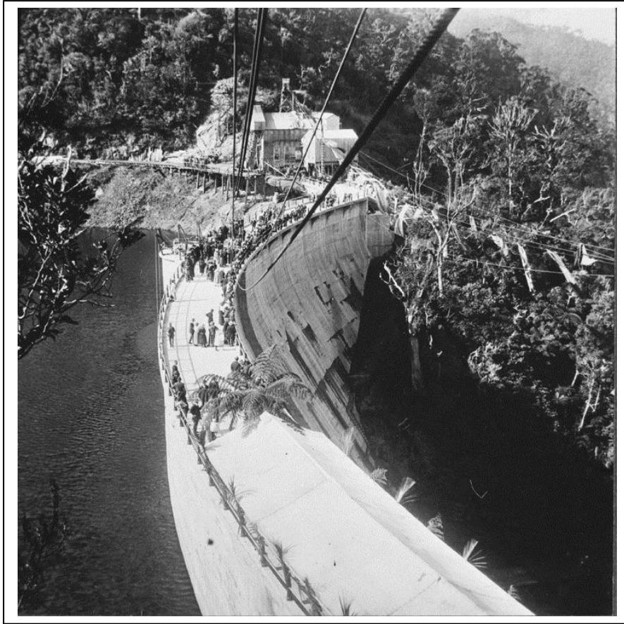
Figure 4: Official opening of the Nihotupu Dam, 1923. Sir George Grey Special Collections, Auckland Libraries, 4-5891
