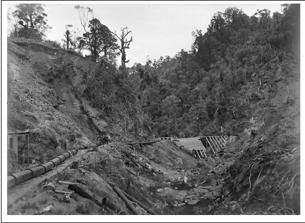
Figure 2: Wooden Dam at Nihotupu in process of demolition, 1914. Sir George Grey Special Collections, Auckland Libraries', 4-2456
