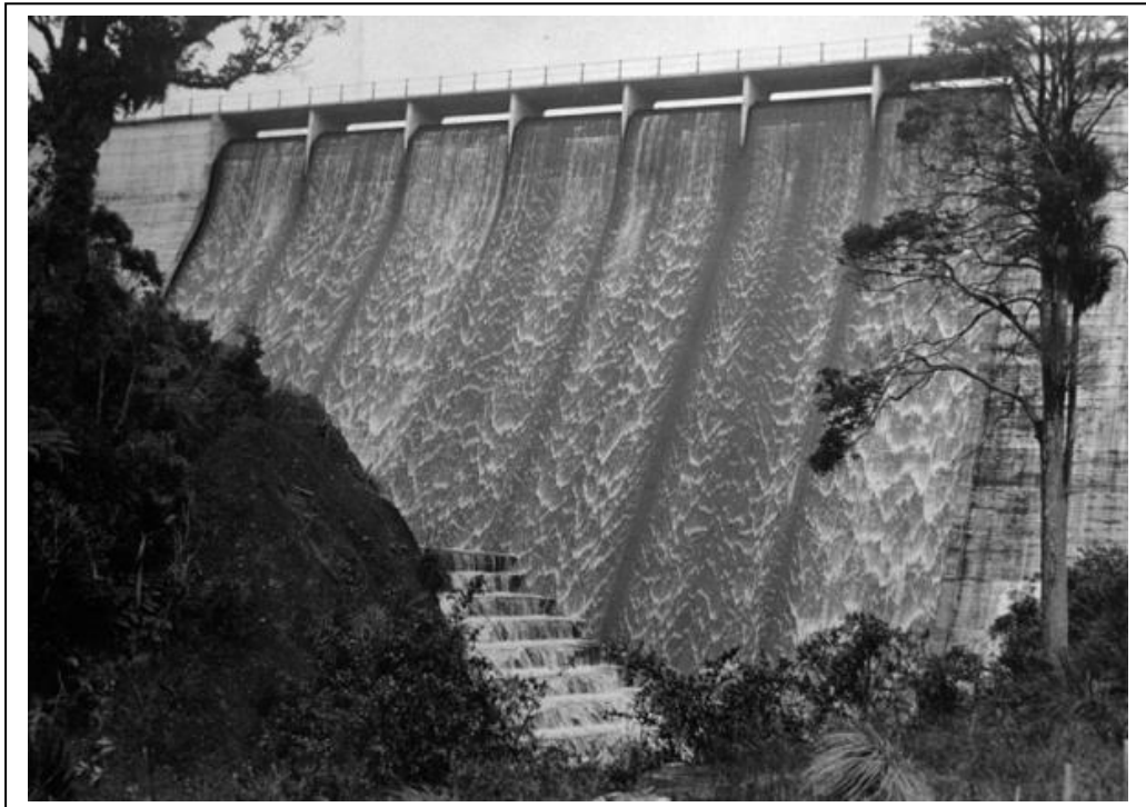
Figure 5: Huia Dam with spillway overflowing. Charles Cecil Roberts, 1933. J. T. Diamond Collection 3913 (7B). Auckland Libraries, West Auckland Research Centre
