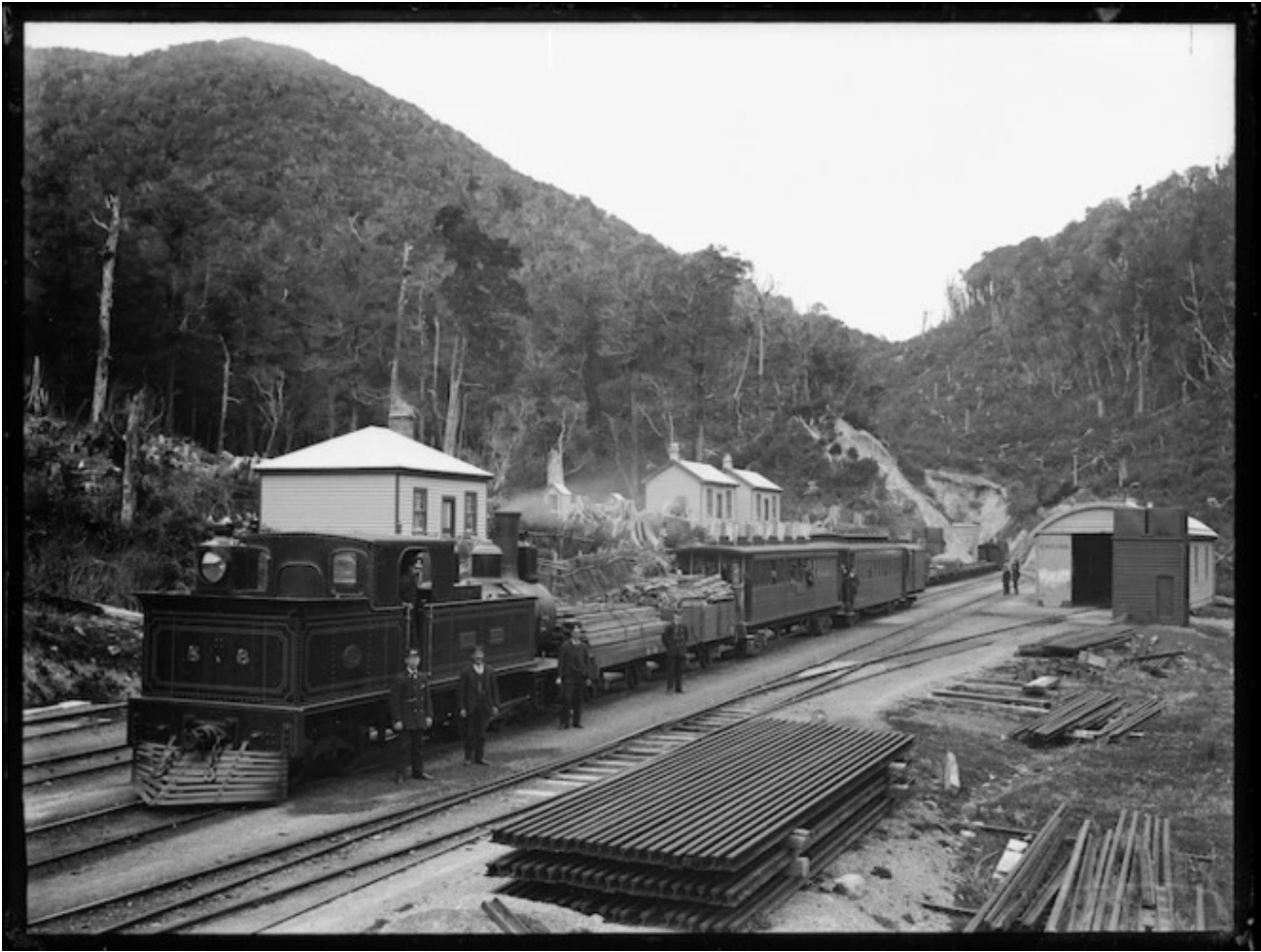
Figure 11: Summit between 1880 and 1890, showing a S class steam locomotive ‘mixed train’ with wagons carrying timber and passengers, about to leave for Wellington, and another train (obscured) being prepared to descend the Incline. Railway workers, including guards J Turner and M Cronin, stand alongside. Note the small number of railway cottages lining the tracks. Photograph taken by William Williams. Ref: 1/1-025480-G, Alexander Turnbull Library, Wellington. https://natlib.govt.nz/records/22699373
