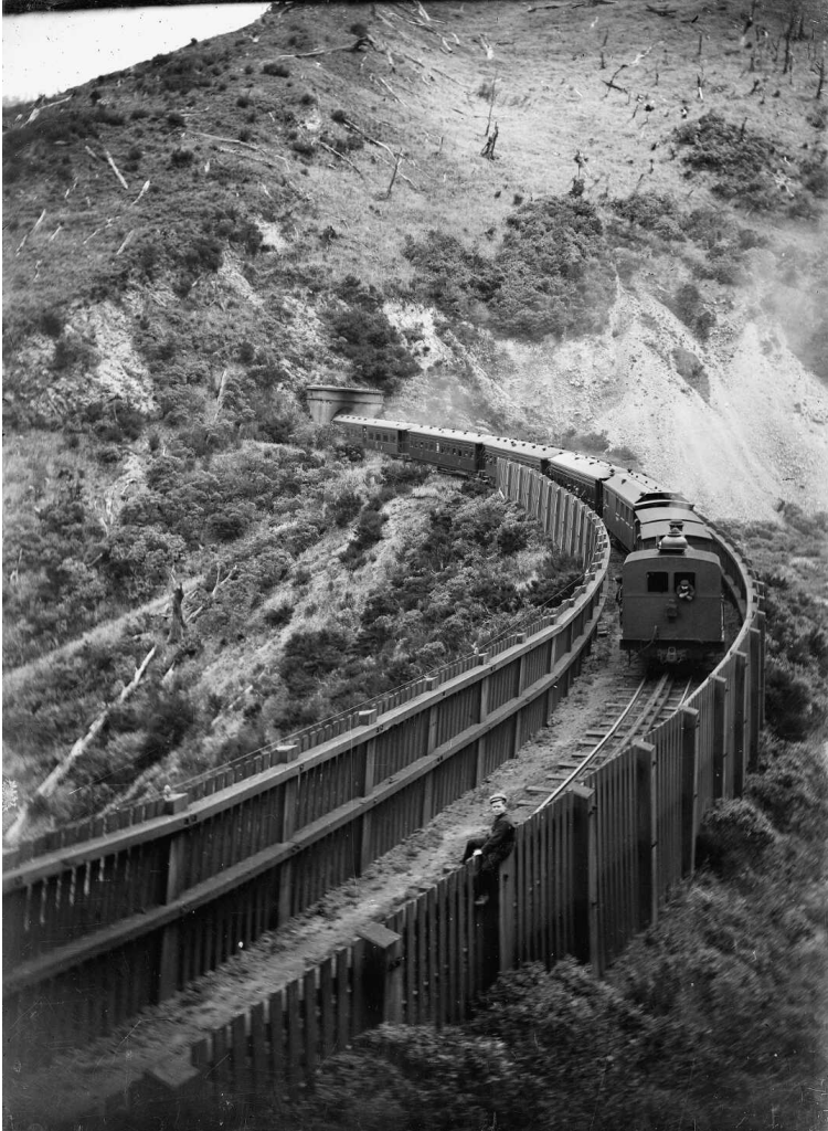
Figure 10: Fell engine and train exiting Siberia Tunnel and passing the windbreaks, ca.1910. Photographer: Albert Percy Godber. Alexander Turnbull Library, Ref: APG-0153-1/2-G. /records/22300820
