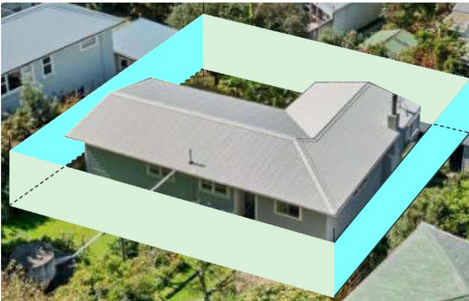
Figure 7: Possible method to measure plan shape at diaphragm levels
