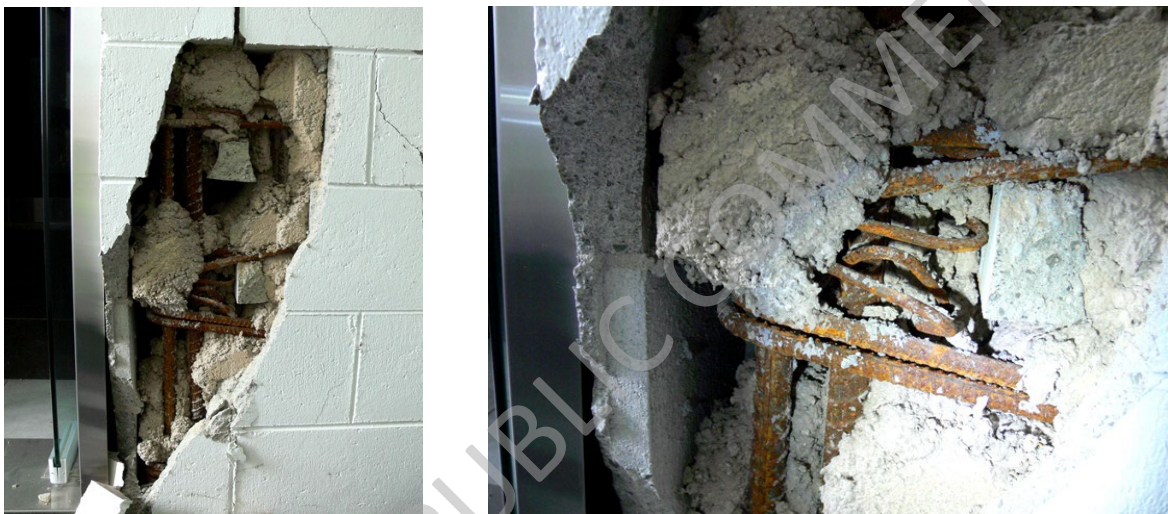
Figure C11.3: Example of partial wall failure due to voids in 'filled' cells. Photo credit: Waipapa Taumata Rau University of Auckland.
