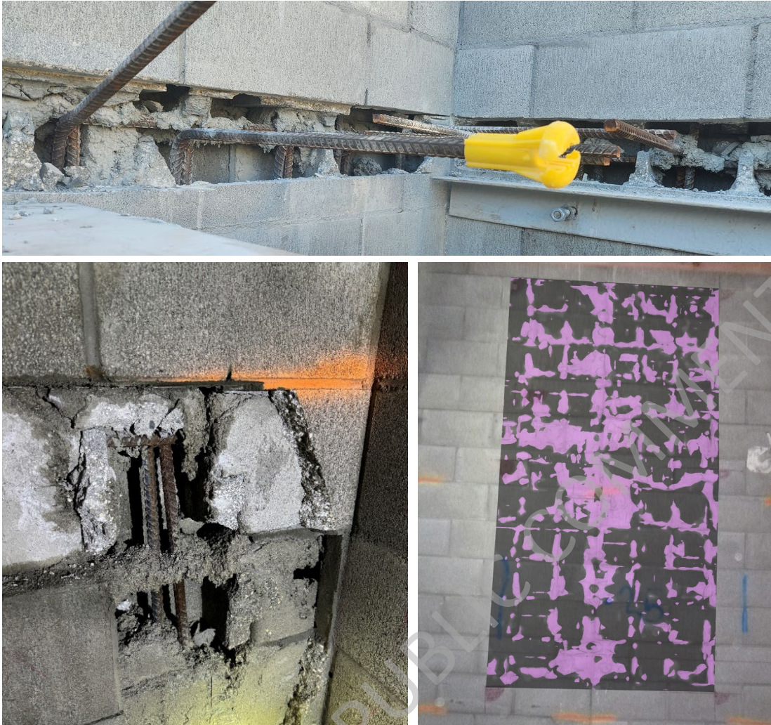
Figure C11.4: Top and Left: Voids discovered in a SED RCM wall, built in 2024. Right: Ground Penetrating Radar scan showing areas of low density. Note only some purple zones are voids, a skilled scanner operator was needed to identify the actual voids in these scans. Photo credit: Beca Ltd
