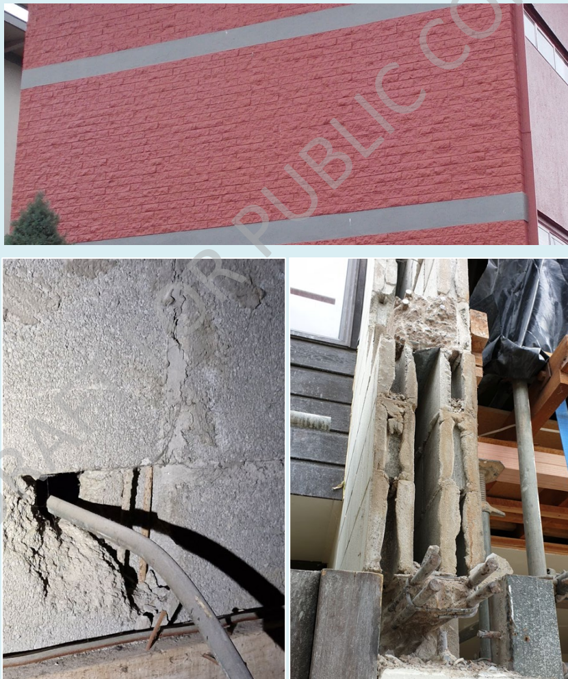
Figure C11.6: Top: 100 mm high concrete blocks made to look like URM. Left: reinforcement in vertical mortar beds. Right: two wythes of 10 series block separated by a cavity with bridging bond beams. Photo credit: Kent Huxford/Lewis Bradford Consulting Engineers
