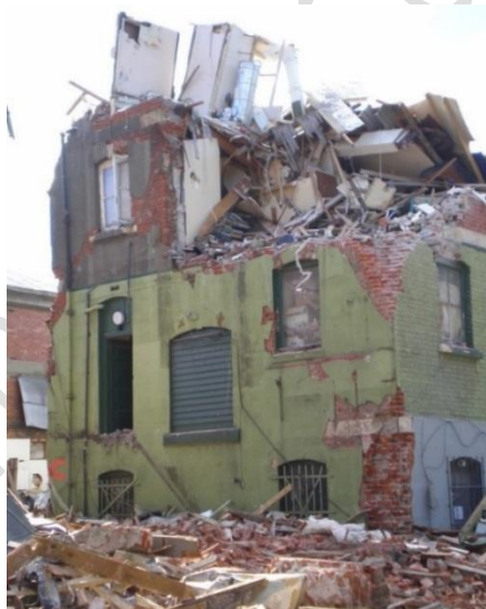
Figure C8.38: Reduction of damage towards base of building as axial load increases (Dunning Thornton)
