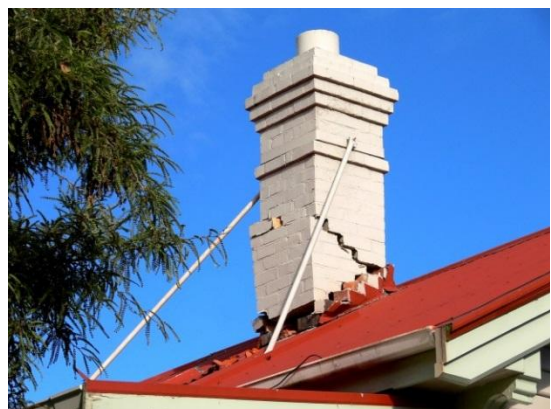
(b) Chimney at onset of falling (Dizhur)
