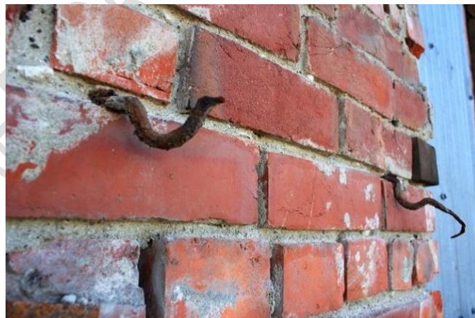
Figure C8.61: Metal cavity ties in rusted condition (Dizhur et al., 2011)
