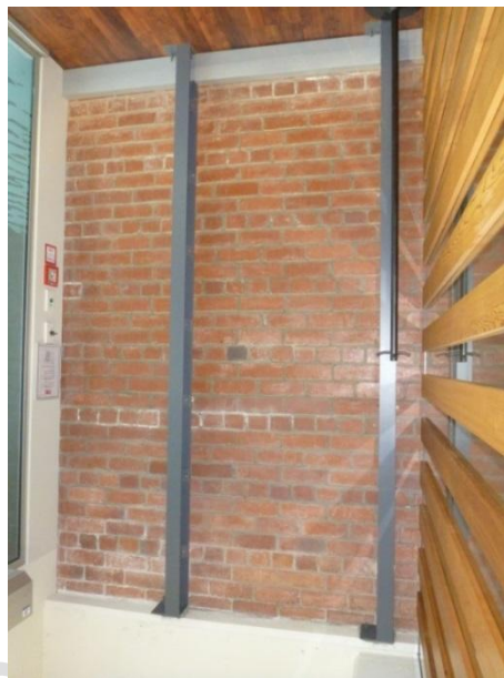
Figure C8.31: Bracing of wall against face load (Dunning Thornton)
