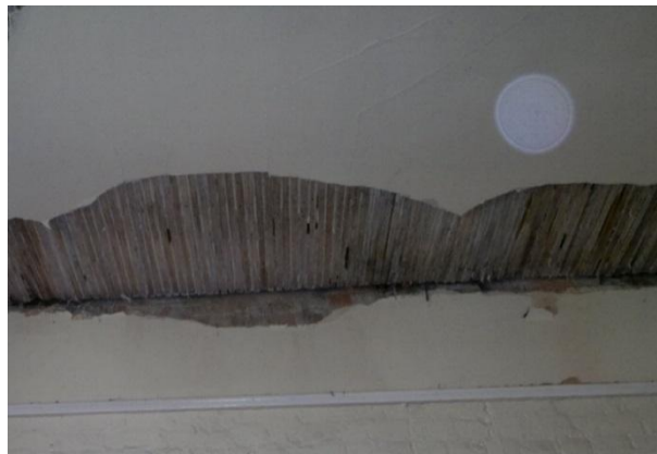
Figure C8.40: Lath and plaster ceiling. Note that stresses where shears are transmitted to the wall have caused the plaster to delaminate from the timber lath
