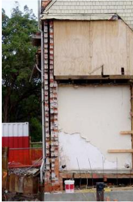
Figure C8.8: Change in cross section of brick wall (Holmes NZ LP)
