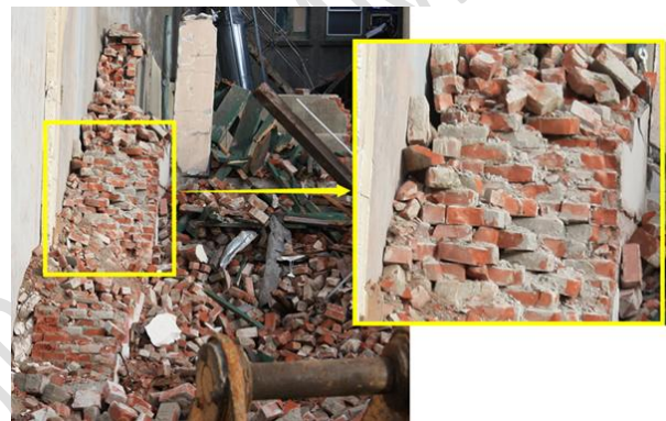
(b) Ground floor of the 7-storey Manchester Courts building demolished after the 2010 Darfield earthquake
