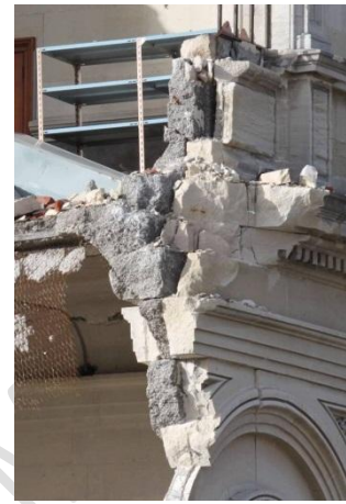
(c) Stone facing and concrete core
