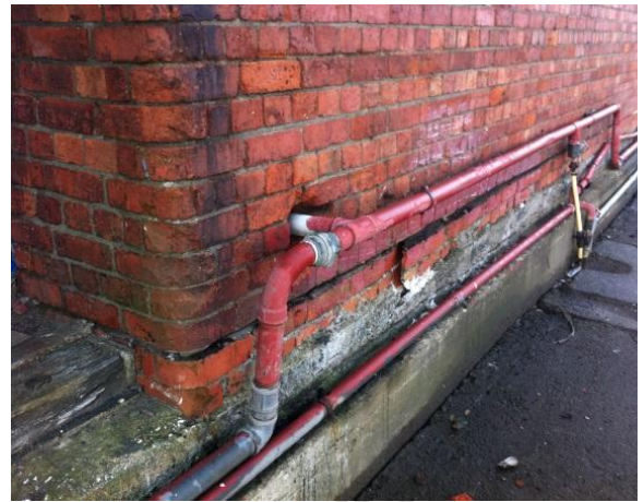
(b) Bitumen DPC and sliding evident after the 2013 Cook Strait earthquakes
