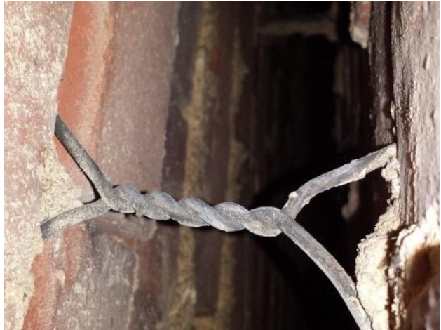
(b) Typical example of cavity observations
