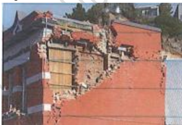
(c) Post-June 2011 event – wall collapse
