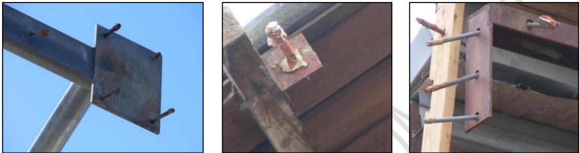
Figure C8.29: Anchor failure from the Canterbury earthquakes (University of Auckland)
