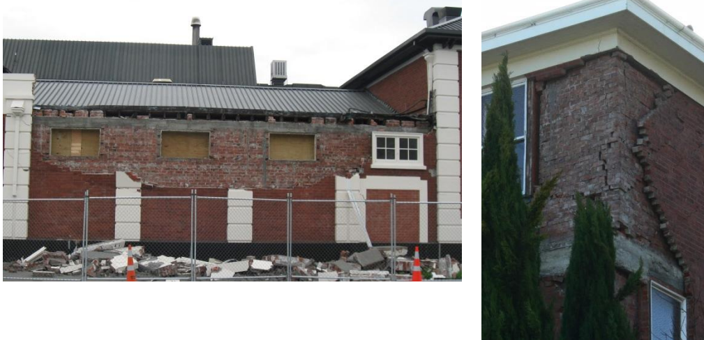
Figure C8.49: Failure of URM cavity walls (Dizhur)
