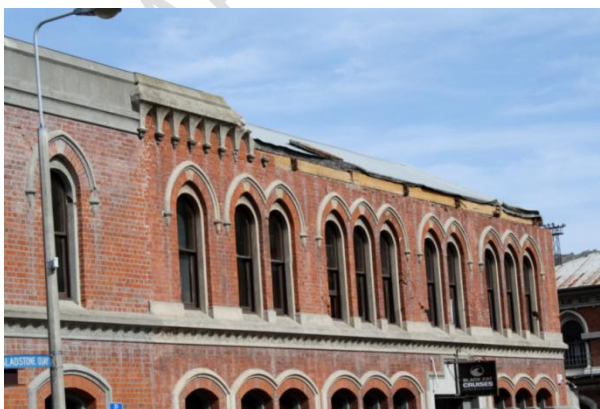
(a) Out-of-plane instability of parapet (Beca)
