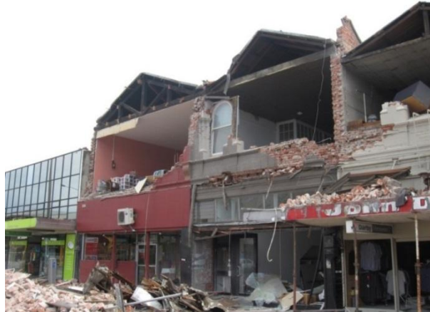
Figure C8.56: Face-load failure of URM façade exacerbated by outward loadings from downward force on canopy. Note the adjacent propped canopy did not collapse. (Dunning Thornton)
