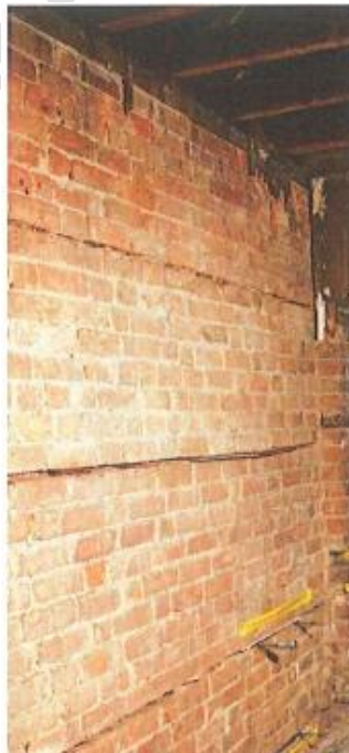
Figure C8.25: 12 mm timber built into every eighth course for fixing linings
