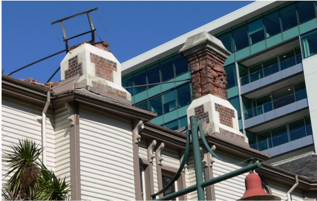
Figure C8.30: Performance of braced chimneys in the Canterbury earthquakes (University of Auckland)
