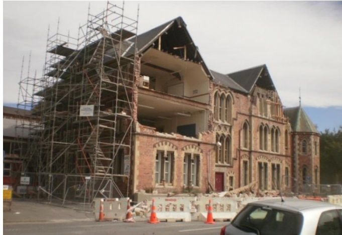
Figure C8.20: A lack of connection of the walls parallel to joist and rafters with diaphragms and return walls leading to collapse of wall due to face loading
