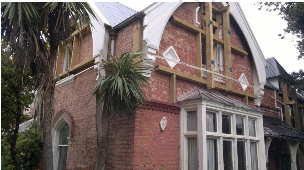
Figure C8.2: Temporary securing of a mildly damaged solid masonry URM building (Dunning Thornton/Heartwood Community)
