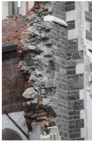
(b) Stone facing and brickwork backing
