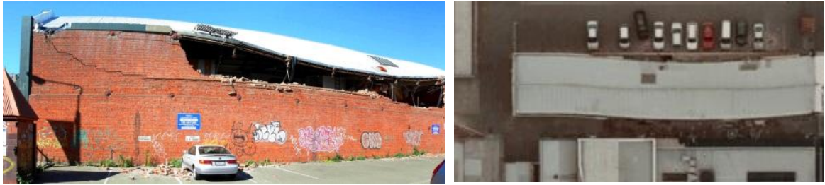
Figure C8.39: Out-of-plane wall failure due to excessive roof diaphragm movement (Dizhur et al., 2011)
