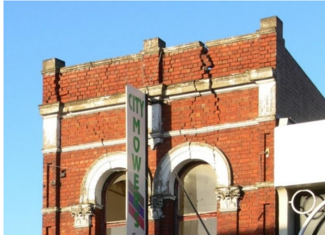
Figure C8.27: The wide cracks through bond beams indicate a lack of reinforcement in the beam (Dizhur)
