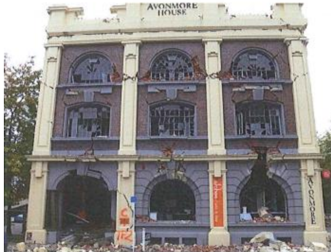
Figure C8.54: Failure of spandrels. Also note rocking of upper piers and corner cracking of the parapet (Dizhur)
