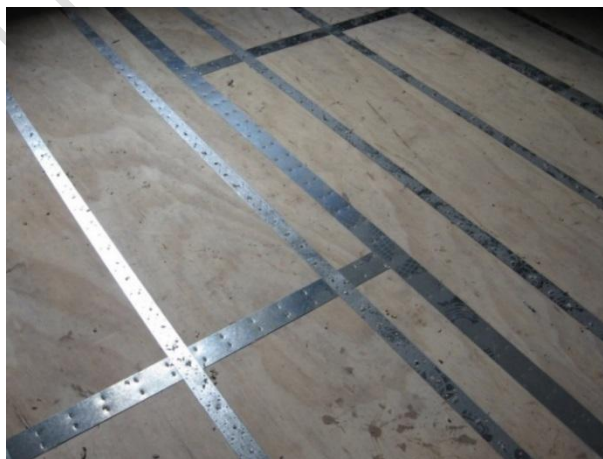
Figure C8.33: New plywood diaphragm (Holmes NZ LP)
