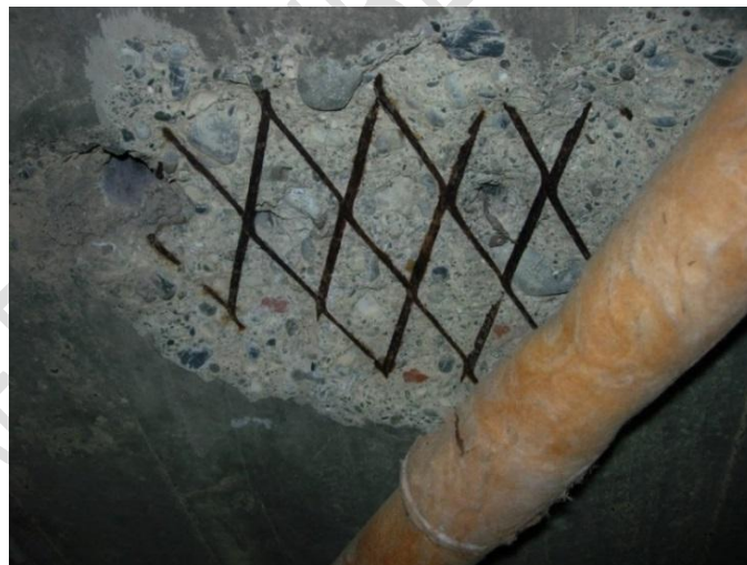
Figure C8.17: Concrete slab with expanded metal lath reinforcement. Corrosion of the lath from carbonation of the concrete over time has caused the concrete to spall
