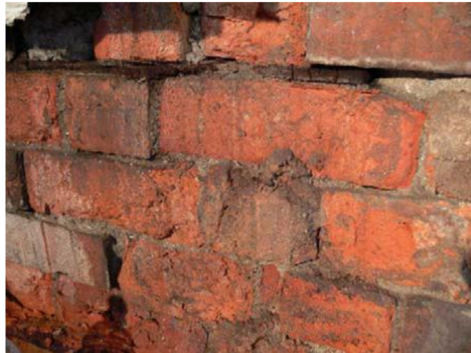
Figure C8.60: Severely degraded bricks and mortar due to moisture ingress (Ingham and Griffith, 2011)
