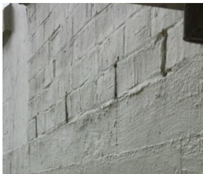
Figure C8.9: Cavity wall indicators (Holmes NZ LP)
