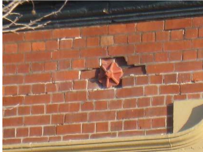
Figure C8.42: Plate anchor on verge of punching shear failure (Dizhur et al., 2011)
