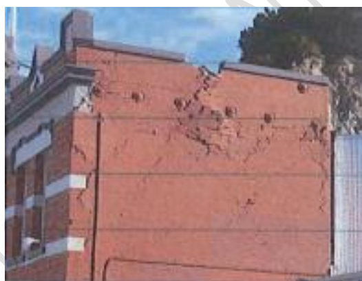
(b) Post-February 2011 event – wall section on verge of failure
