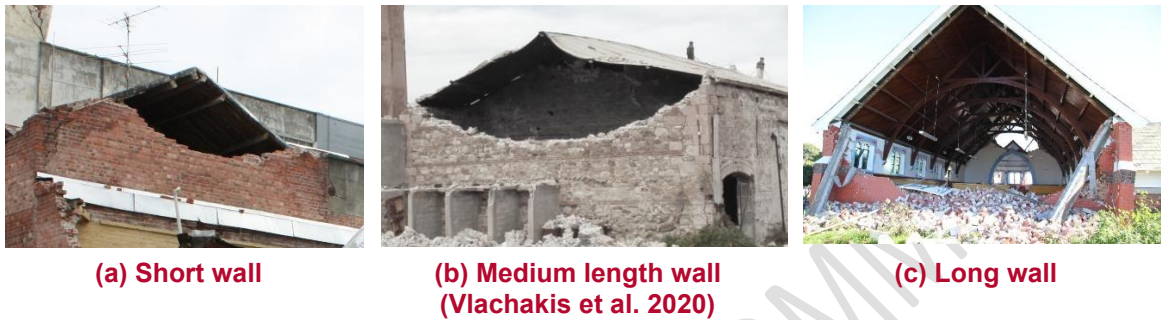
Figure C8.75: Vertical-horizontal spanning gables failure mechanism
