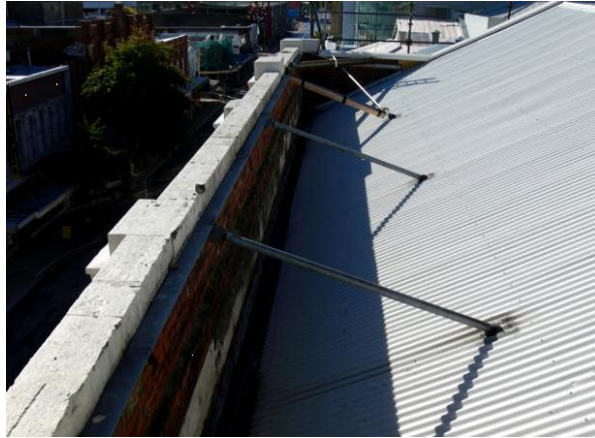
Figure C8.35: Parapet bracing. Note a lack of vertical tie-up of the parapet (Dizhur)
