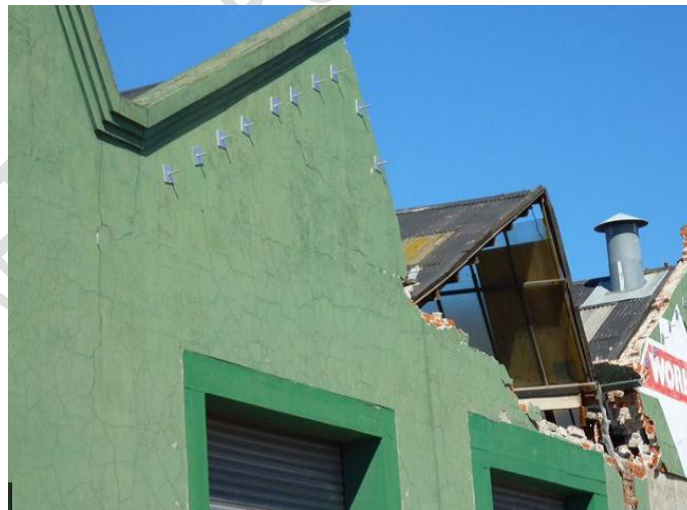
Figure C8.48: Collapse of gable wall. Note a secured gable end that survived earthquake loading and a companion failed gable end that was not secured (Ingham and Griffith, 2011)
