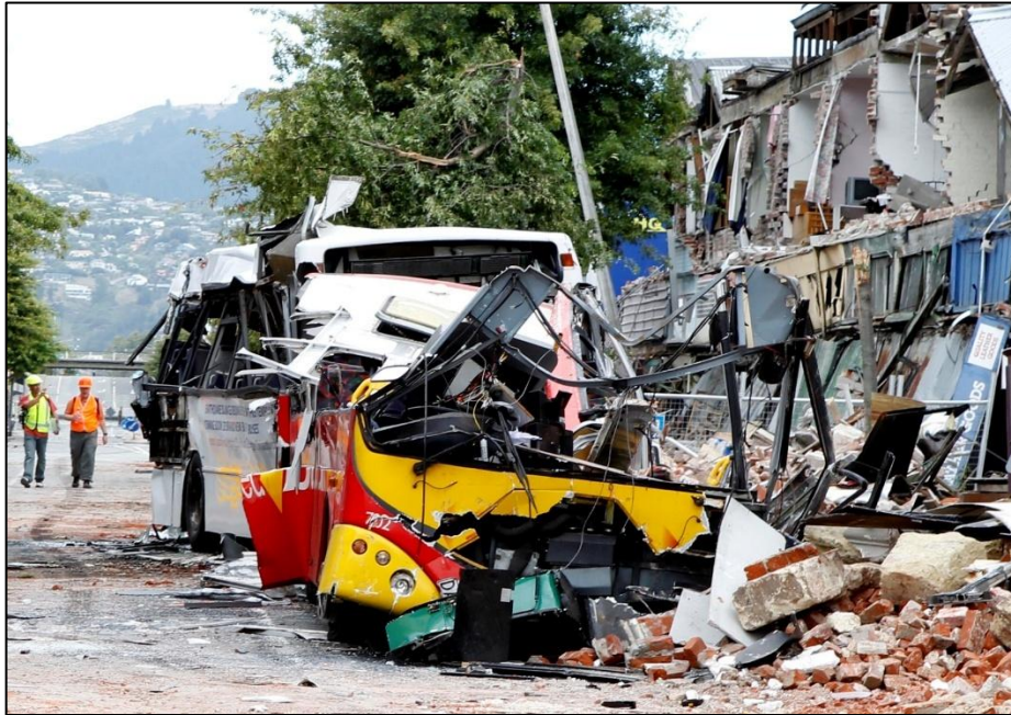
Figure C8.1: Collapsed masonry façade causing fatalities in the Canterbury earthquakes
