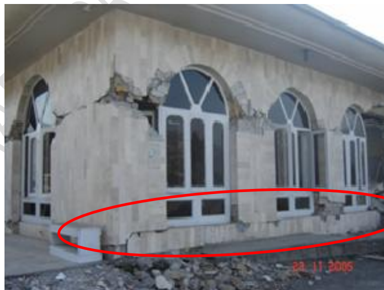
Figure C8.51: Rocking and delamination of bricks of a one-storey unreinforced brick masonry building with reinforced concrete roof slab (Bothara and Hıçyılmaz, 2008)
