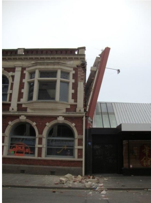
Figure C8.47: Out-of-plane instability of wall under face load due to a lack of ties between the face-loaded wall and the rest of the structure (Sharpe)
