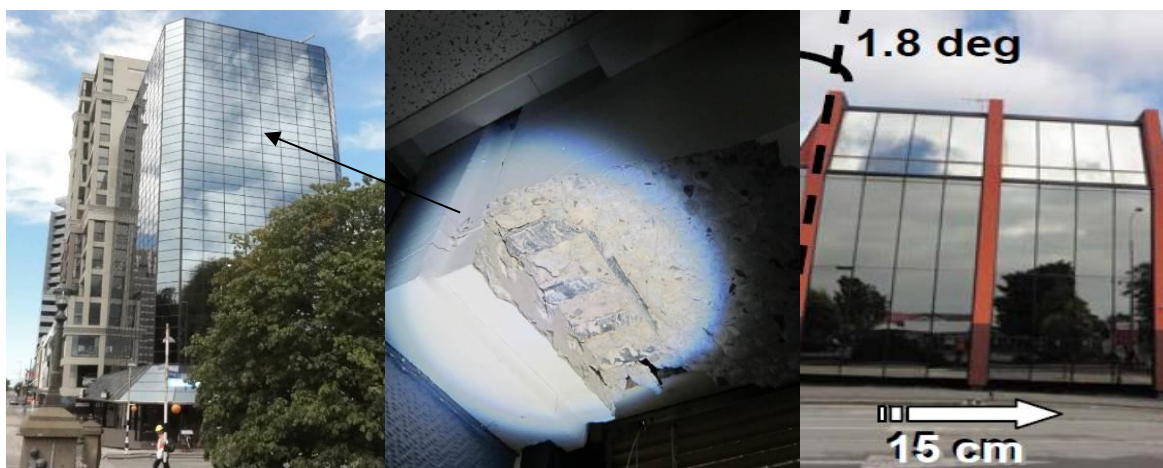
(a)-(b) 1980s high rise on basement and raft foundation; with beam plastic hinges observed throughout the building
