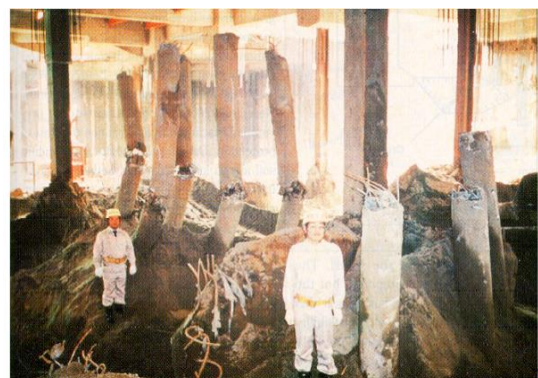
(b) Pile shear failure observed in an excavation 20 years after the Niigata 1964 earthquake
