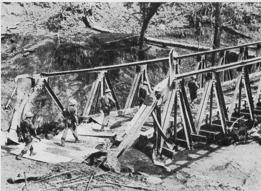
Single-tress army-type road bridge 12 ft. wide by 80 ft. span, damaged but not destroyed by the Japanese. Such bridges were widely used in this theatre of war.
