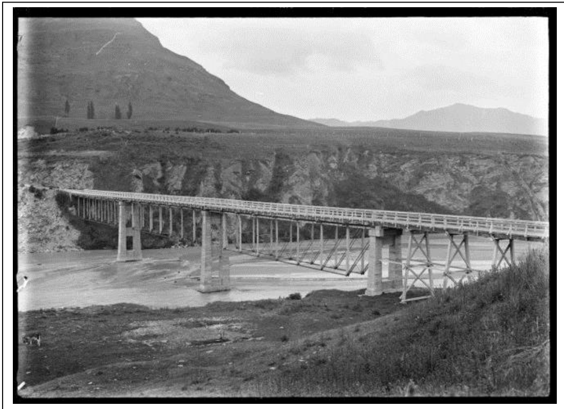
Bridge over the Shotover River in the Lower Shotover area, 1926. Godber, Albert Percy, 1875–1949: Collection of albums, prints and negatives. Ref: APG-1683-1/2-G. Alexander Turnbull Library, Wellington, New Zealand. http://natlib.govt.nz/records/22806436
