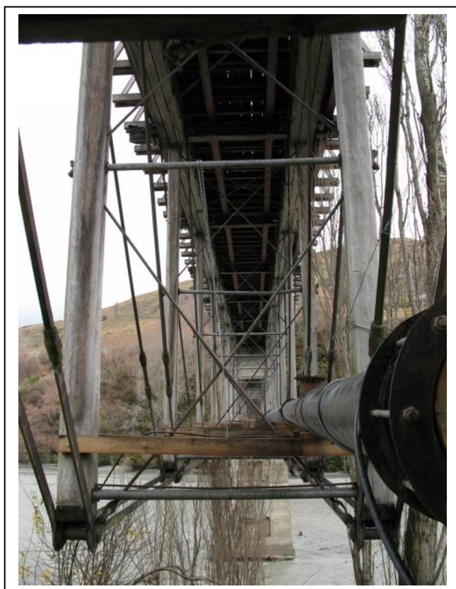
View through trusses, Shotover River Bridge, 2011. Image courtesy of L. Smith.
