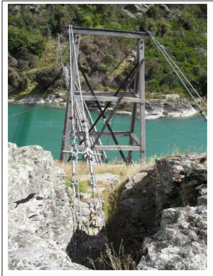
Figure 3: Anchorage of catenary cables, 2011. Photograph courtesy of J. Dee.
