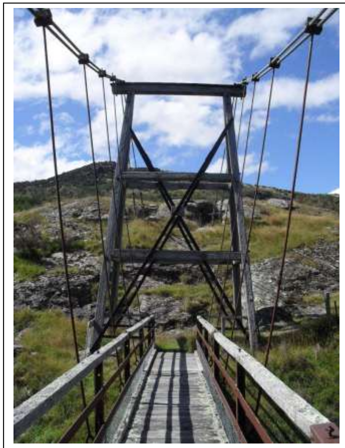
Figure 2: Timber A-frame towers of the suspension bridge, 2011. Photograph courtesy of J. Dee
