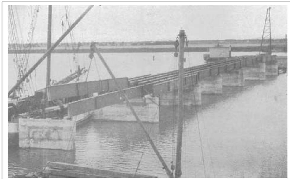
**Figure 1:** Construction of the Kopu Bridge. *Appendix to the Journals of the House of Representatives*, Wellington, 1927, Vol. II, D-1
