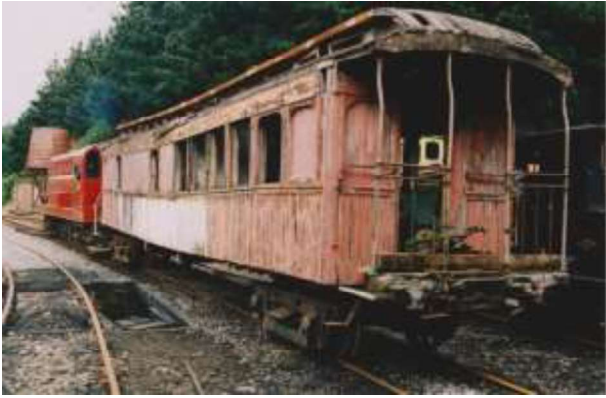
Figure 4: WMR No. 52 being transported to the project workshop. The body sags after removal of truss rods and much rot is apparent.
