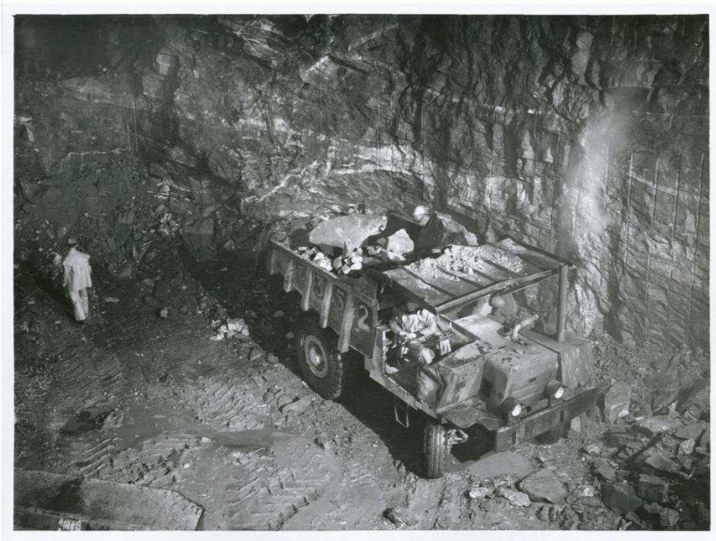
Above: Removing rubble from the machine hall, August 1967. Archives New Zealand, R24730709, photographer: Mr Neill.
