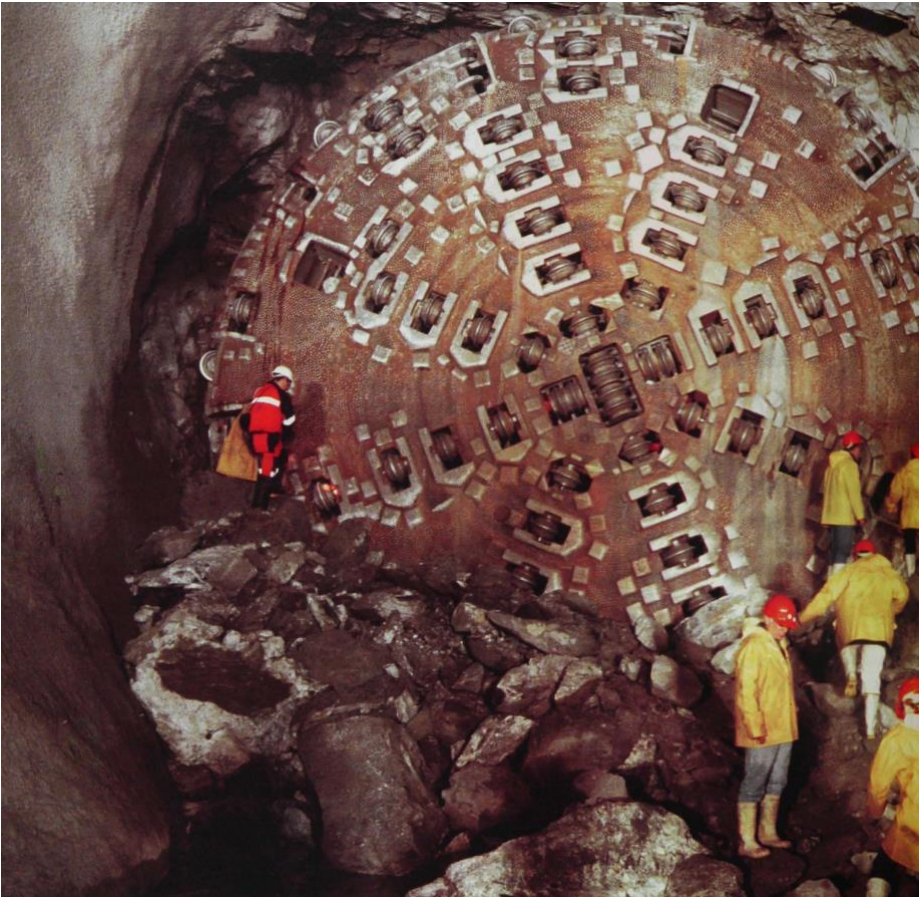
Above: The Tunnel Boring Machine. Photo (cropped): Meridian.
