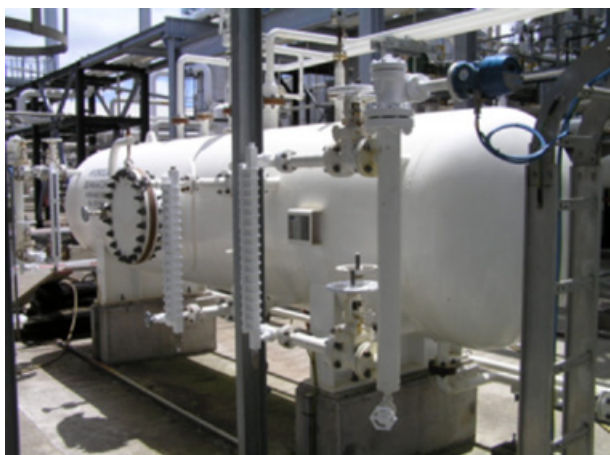
Figure 1. Horizontal pressure vessel on short pedestals
