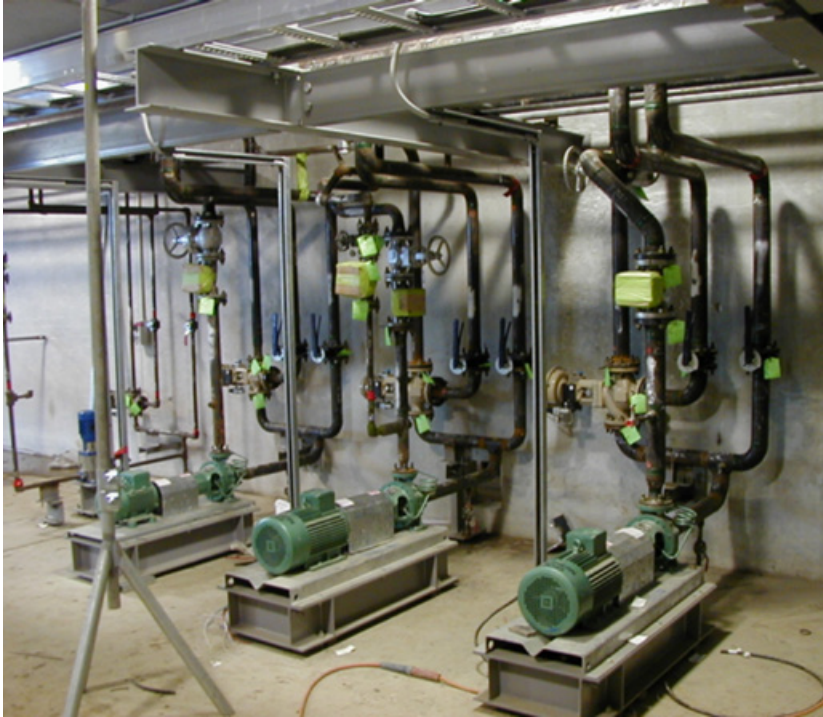
Figure 5: Rigid structures – pumps skid mounted at grade.
