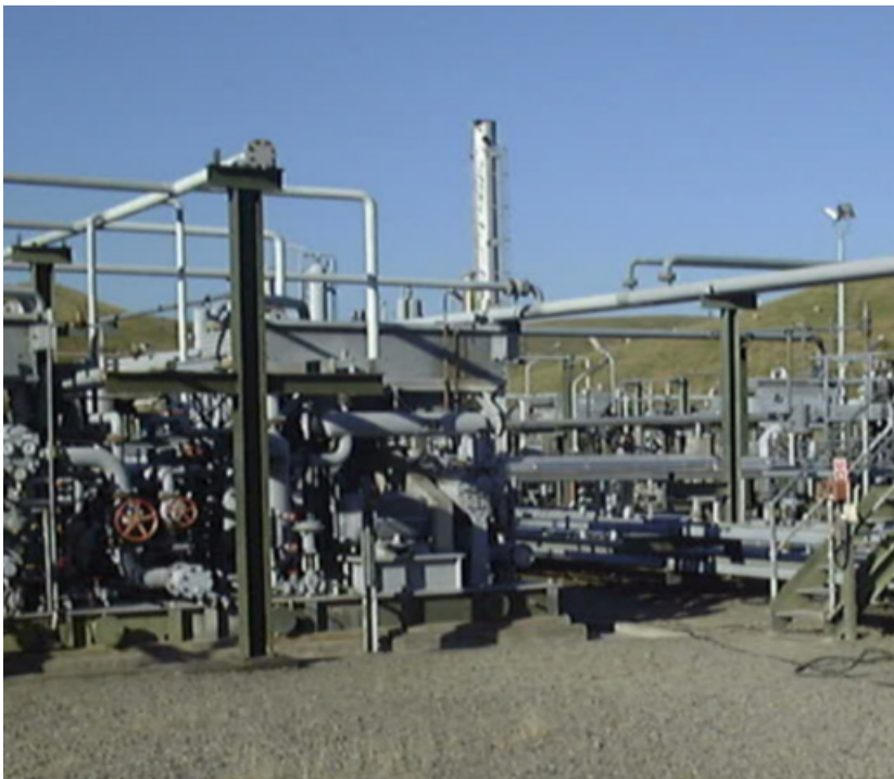
Figure 12: Pipes and pipe supports.
