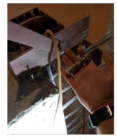
This connection cannot transfer the loads required & is not a recommended detail
