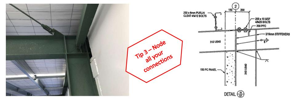
Eccentric connection and indirect load path from tension brace to the strut
