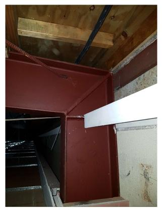
Eccentric connection from bracing, relying on indirect load paths to transfer from tension brace to the PFC collector This connection and member cannot transfer the required forces
