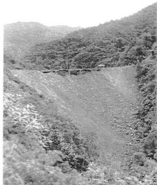
Fig. 5 30m Filling at Wharekakaho
