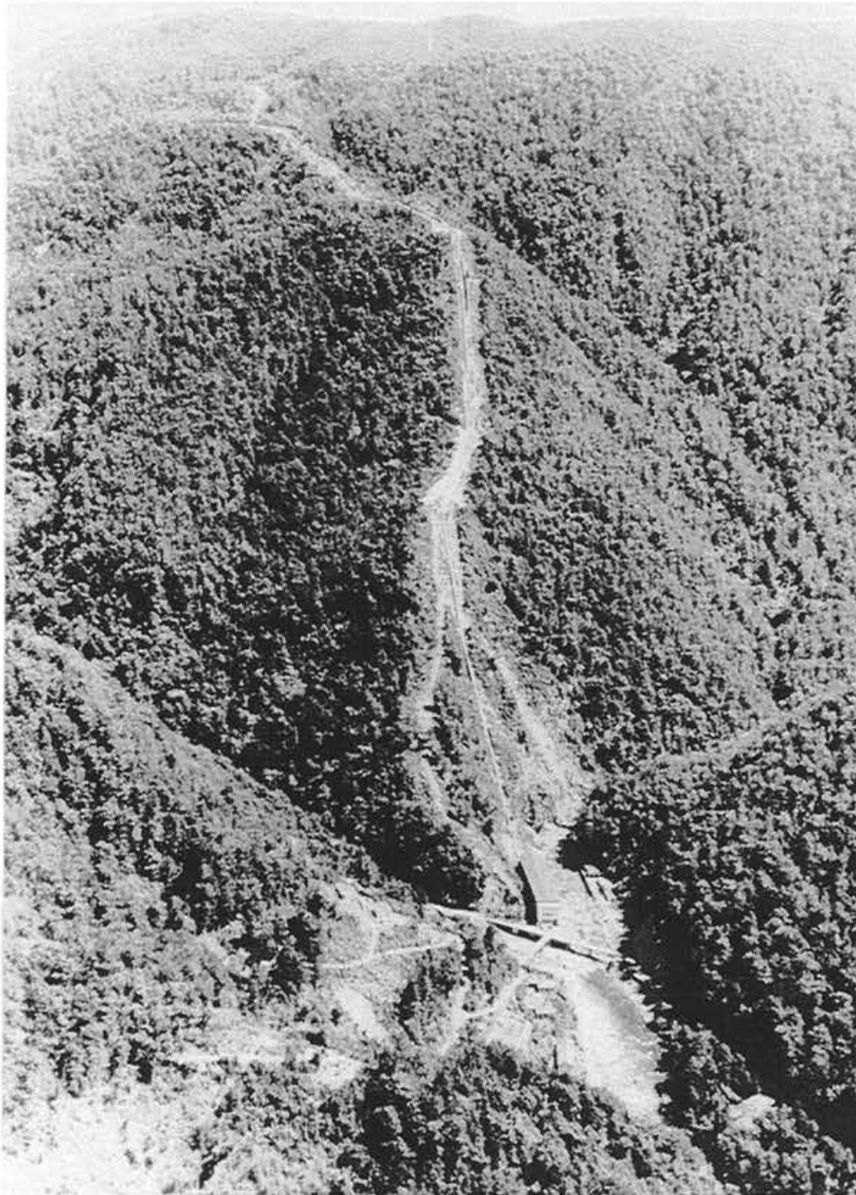
Fig. 6 1955, Station at full 32 MW power with second penstock and new powerhouse. Road to dam left, Takaka right, and village in foreground. (ECNZ)
