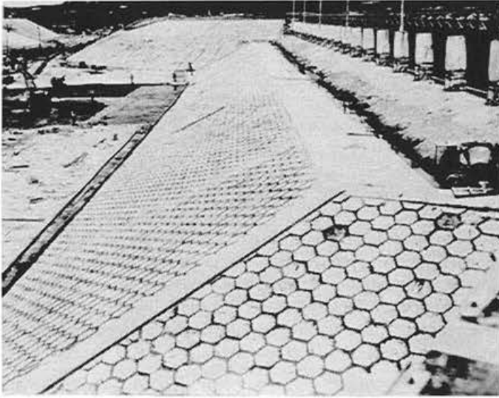
Fig. 4 Hexagonal Slabs of The Forebay Lining
