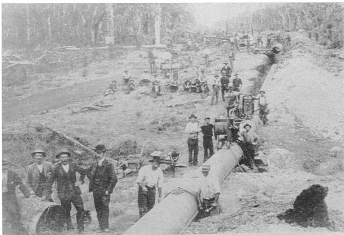
Coolgardie Water Supply: Pipe caulking machine.
