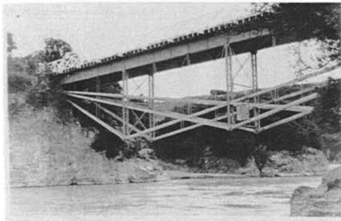
Ironwork Rakaia Gorge Bridge
