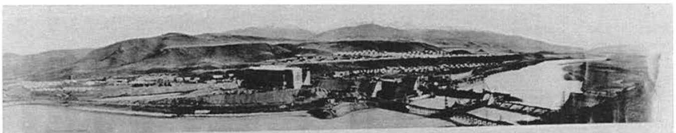
Fig. 7 Waitaki Powerhouse and Central Dam Pier
