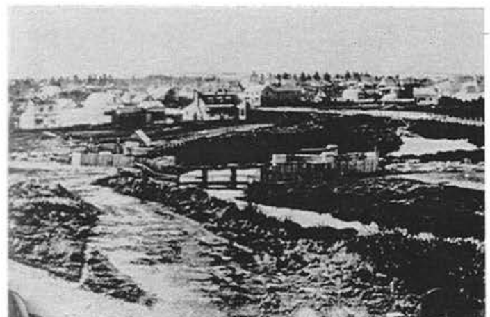
Figure 2. Building the Bridge Foundations 1864 - Dr A.C.Barker (courtesy Canterbury Museum)
