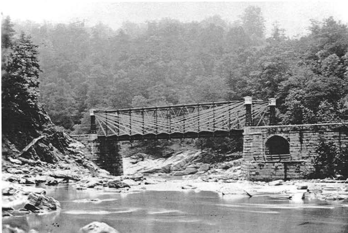
Patapsco River Crossing of B and O, Maryland, Bollman through truss c, 1869 (photograph B and O collection Museum of History and Technology Smithsonian Institution, Washington D.C.).
