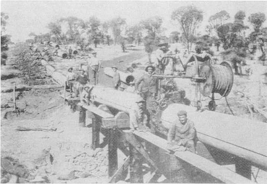
Coolgardie Water Supply: Pipe caulking machine specially invented for the scheme.
