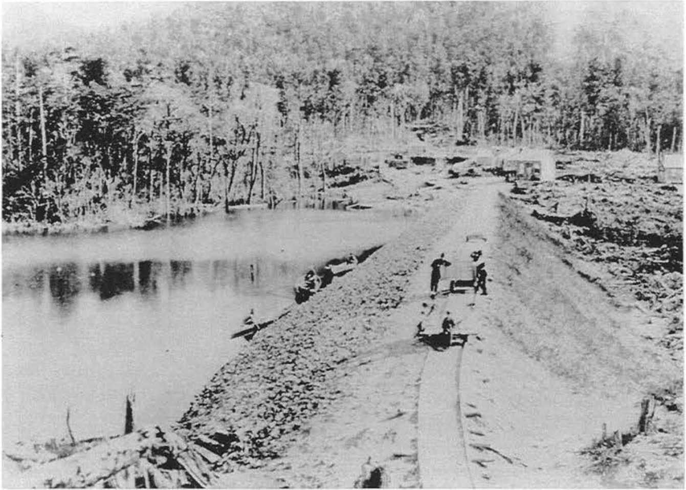
Headworks, Nelson Creek water race, Lake Hochstetter. Photo by W.H. Perkins, courtesy of Canterbury Museum, Christchurch, N.Z. (ref. 2023)
