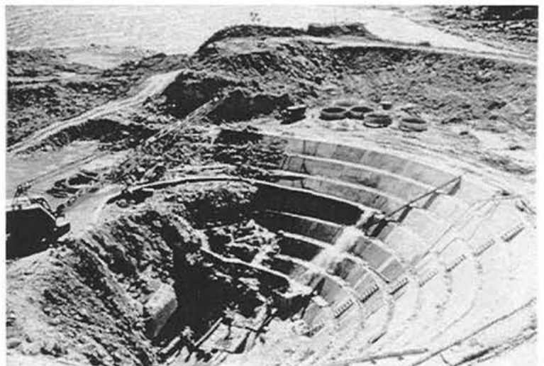
Fig. 6 The Kaitawa Intake Structure Under Construction
