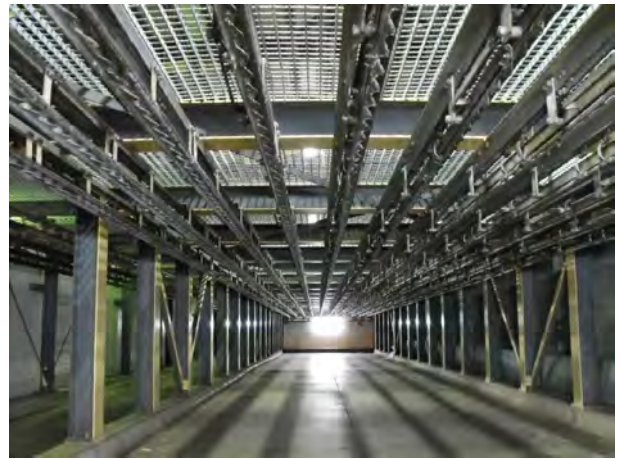
Figure 4: Typical modern air-blast carcass freezer
