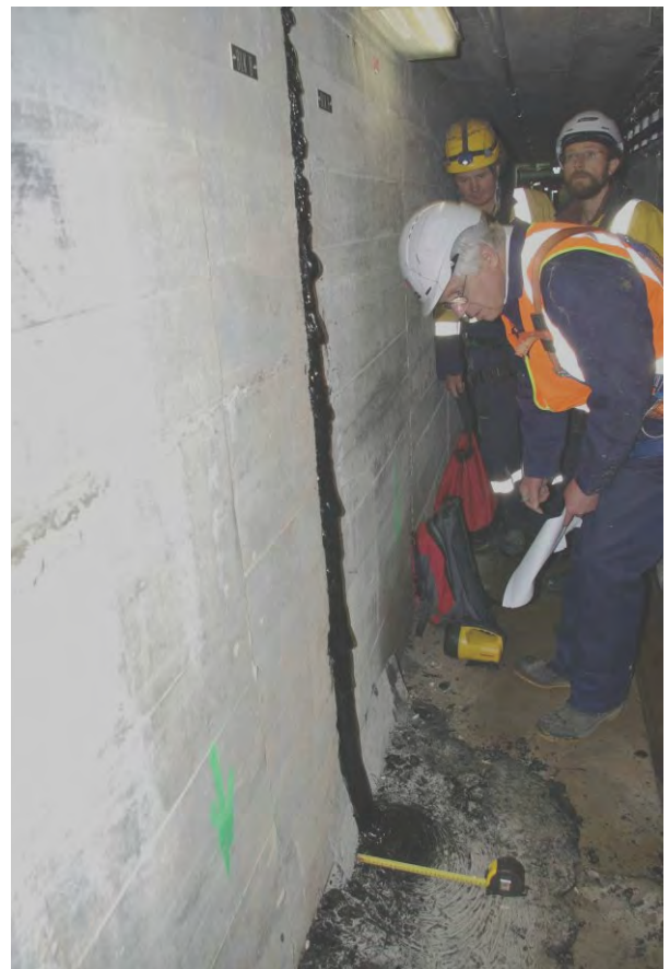
Figure 30. Bitumen water-stop extruding into middle gallery
