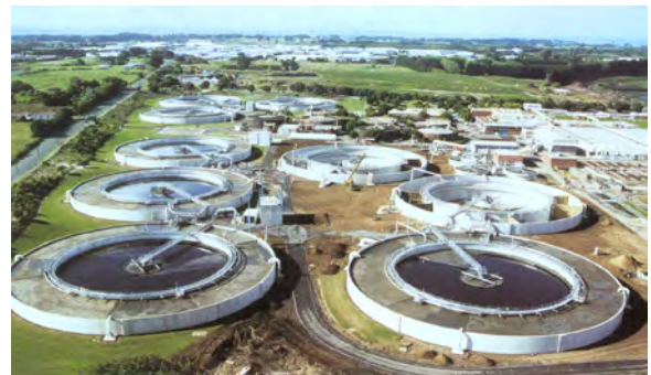
Figure 9. Reactor-Clarifiers –Watercare photo
