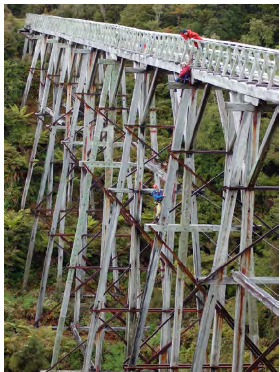
Figure 4. Close inspection of Percy Burn Viaduct piers
