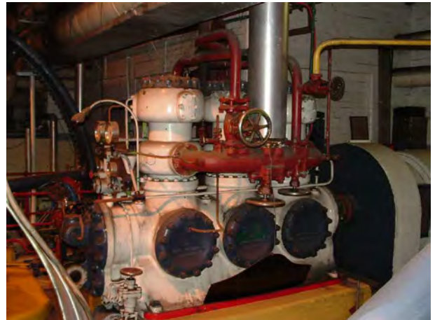
Figure 7: A typical vertical cylinder compressor with enclosed crankcase.
