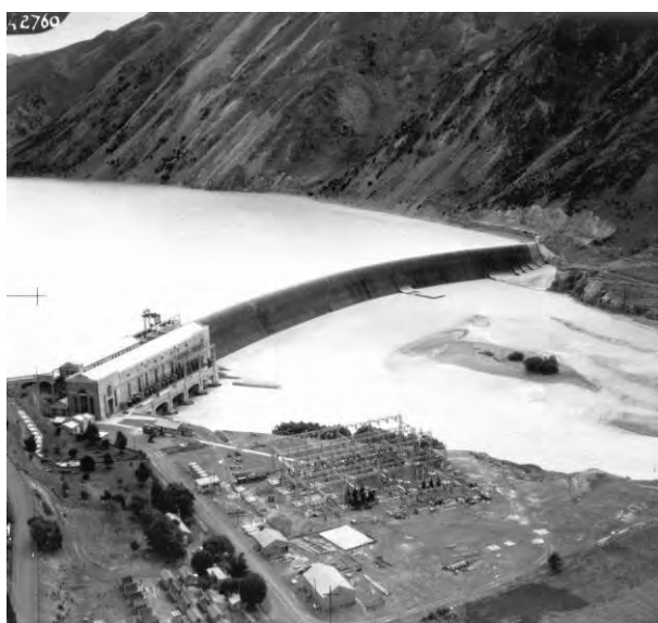
Figure 27. The completed scheme including the original weir and pool fish ladder visible at the end of the power house.
