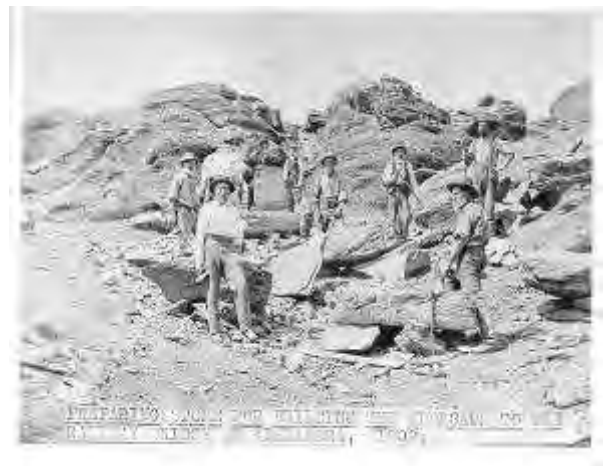
Figure 3. Stonemasons at work cutting stone for another Otago Central Railway bridge - Hocken Library
