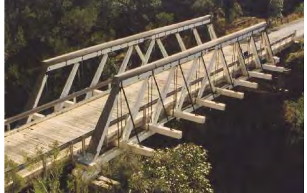
Allan (Howe) normal half-through timber truss bridge
