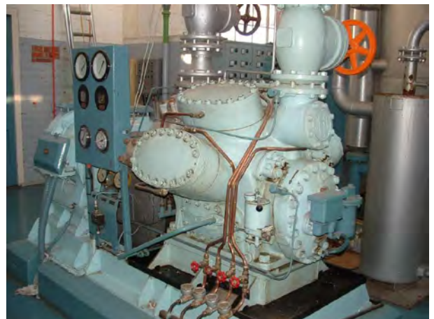
Figure 8: A typical Vee block compressor used both within and outside the meat industry.
