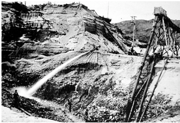
Figure 14. Sluicing and elevating at Roxburgh East using water from Ewings Race
