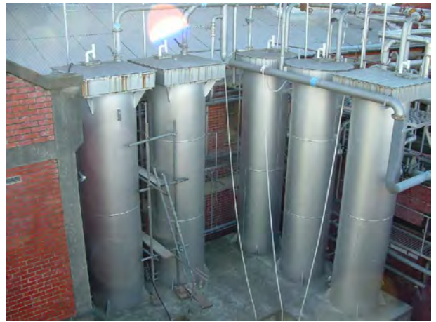
Figure 11: Typical vertical shell and tube condensers used in the meat industry.
