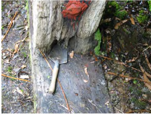
Figure 5. End rot at the ends of pier columns
