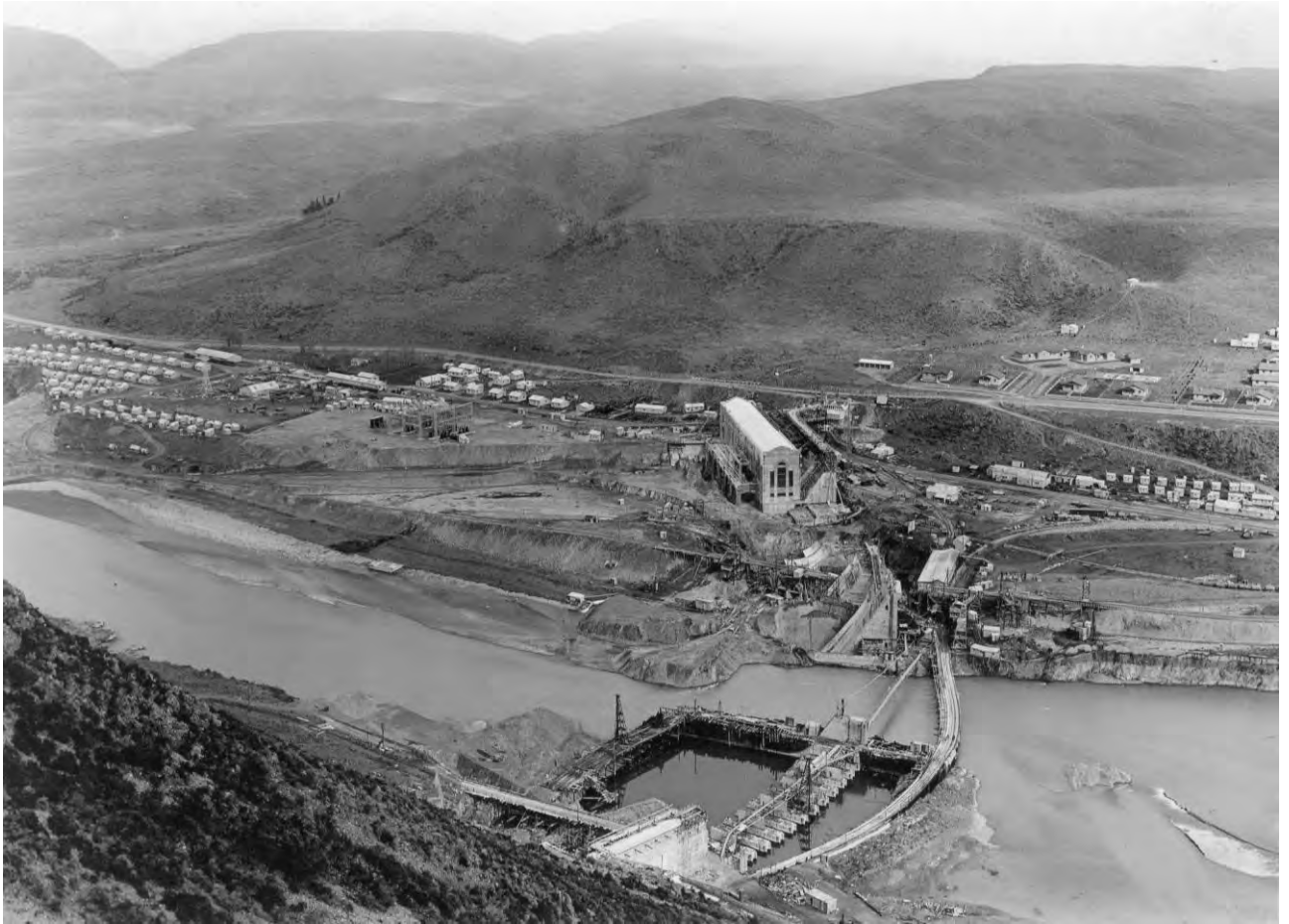
Figure 17. Overall site view from Canterbury abutment before diversion. Switchyard progressing on far bank.
