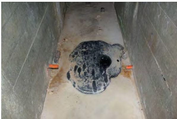
Figure 32. Bitumen infill extruding from diversion sluice
