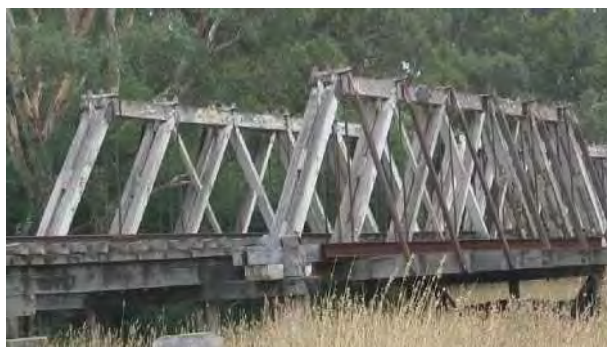
Figure 6. A timber Howe truss railway bridge 1909
