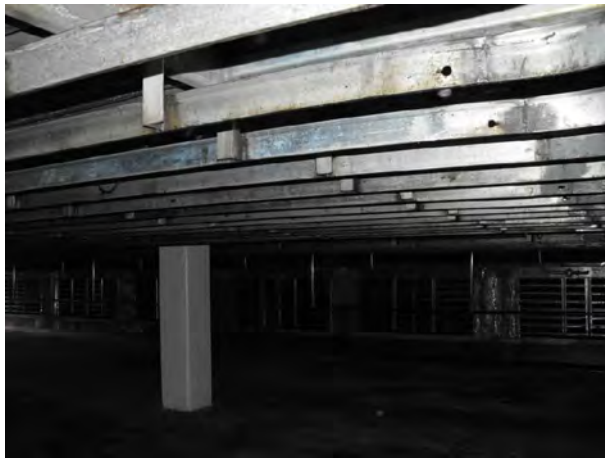
Figure 3: Cross-flow air-blast carcass freezer
