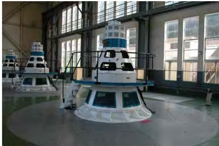
Figure 4. Tungatinah Power Station, the turbine has been rebuilt within the existing chamber and casing, retaining the appearance but not the fabric.
