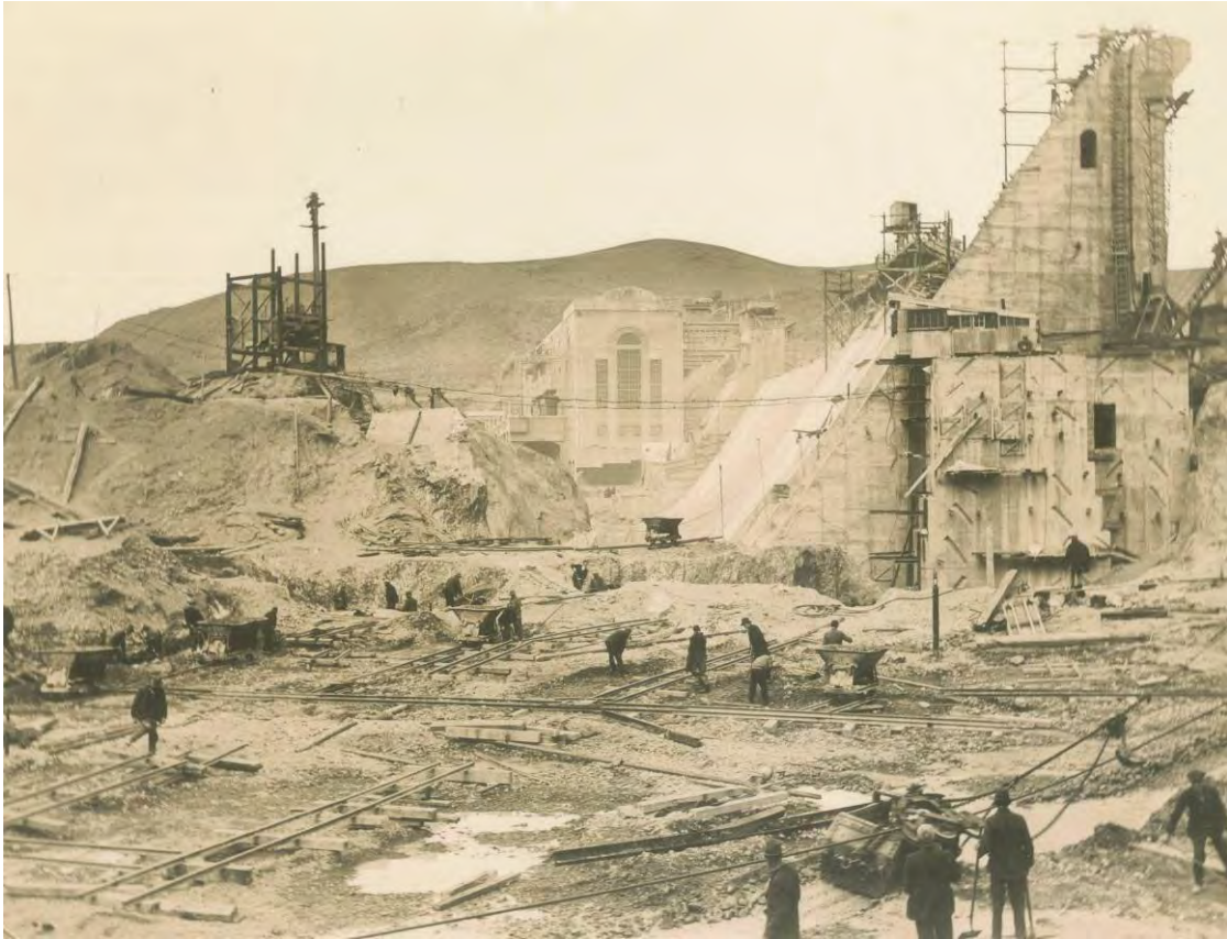
Figure 22. Foundation preparation within Otago coffer dam area c1933. Middle gallery and air gallery visible. Light rail tracks were used extensively for spoil removal, and a dragline is visible in the foreground. However, much of the work involved hard physical labour rather than mechanised techniques in this era.
