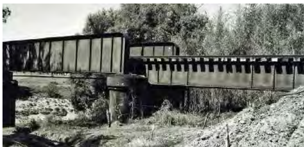
20 m Plate web girder, left [Figure 12 continues]
