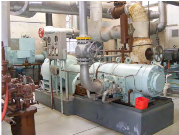
Figure 9: A typical rotary vane booster compressor.
