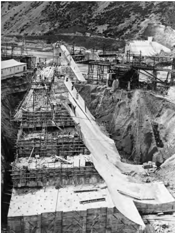
Figure 14. View from Otago bank, block shear keys shown.
