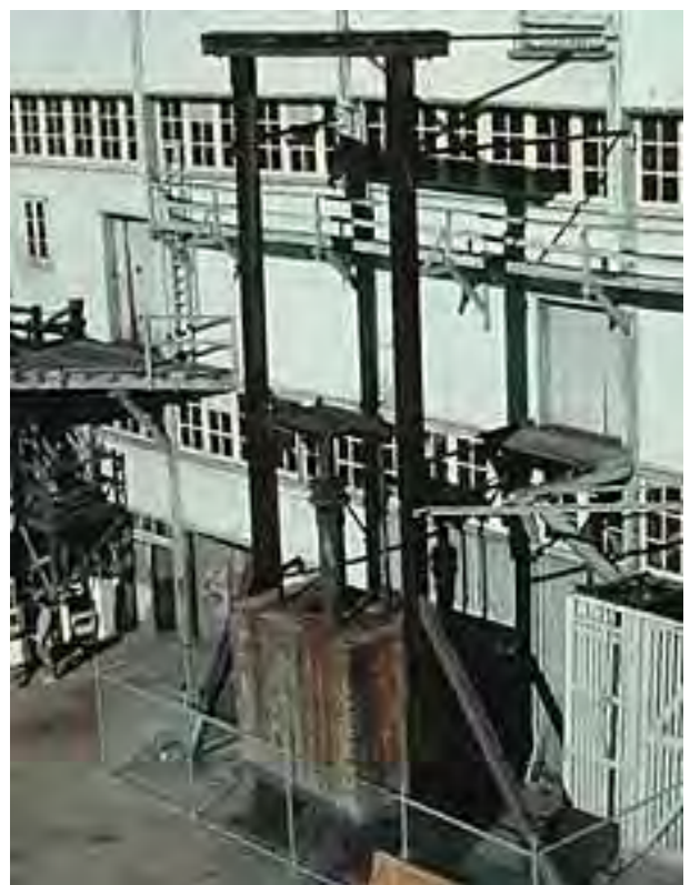
Figure 8. In situ Accumulator, Walsh Bay, Sydney. (Photo – M Doring)
