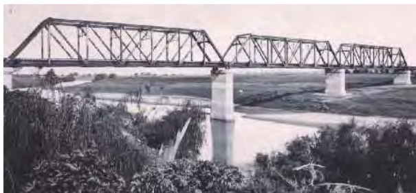
48 m trusses over Hunter River
