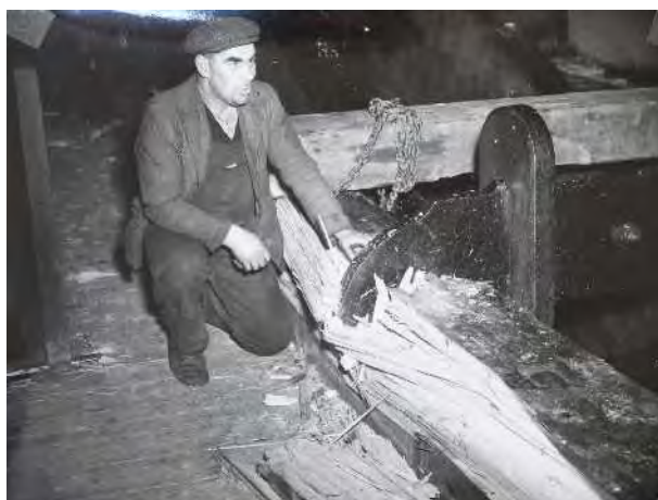
Figure 6. Smashed spring beam
