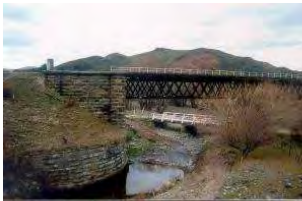
Figure 8. The Capburn Bridge at Tiroiti showing fine stone work abutments and lattice sub structure.
