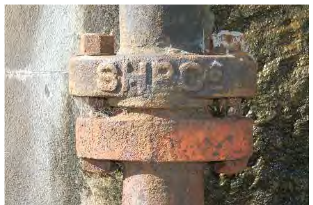
Figure 21. HP Joint on Remnant 4” Main, Sydney.
