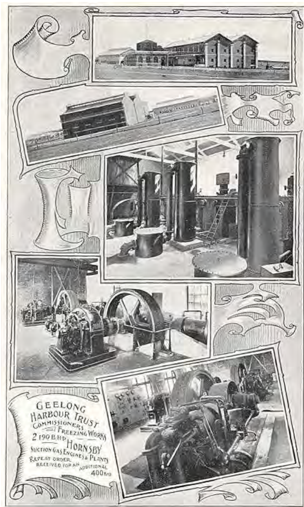
Figure 10: R. Hornsby & Sons Suction Gas Plant at the Geelong Harbour Trust Freezing Works. Powering refrigeration plant for country meatworks, dairy factories and fruit coolstores represented almost a quarter of all Hornsby suction gas sales up to 1915.
