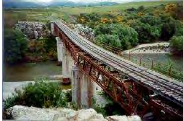
Figure 11. Manuherikia No. 1 bridge was the first built using concrete for the piers.
