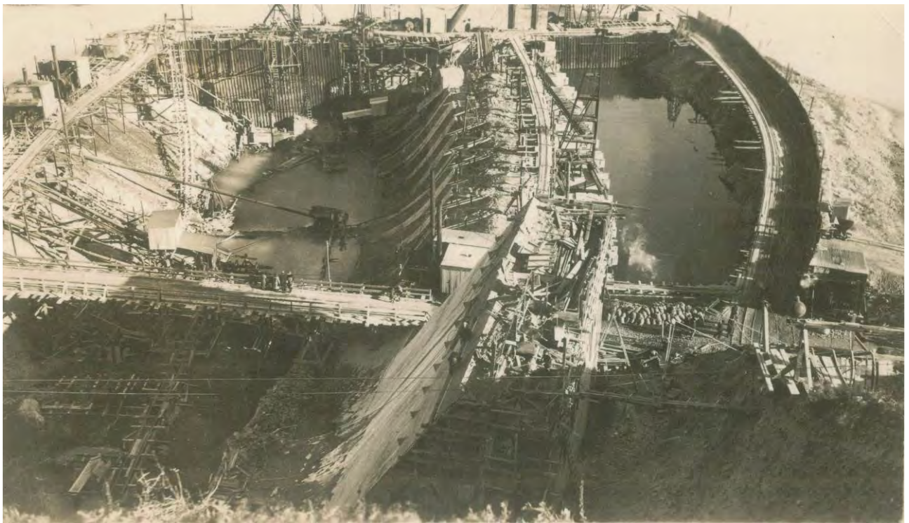
Figure 12. View from Canterbury abutment; blocks progressing adjacent to diversion sluices
