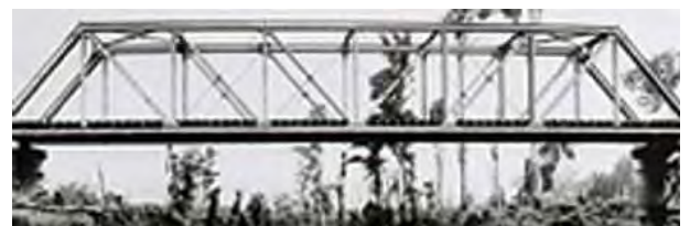
Figure 4. An American steel Pratt truss
