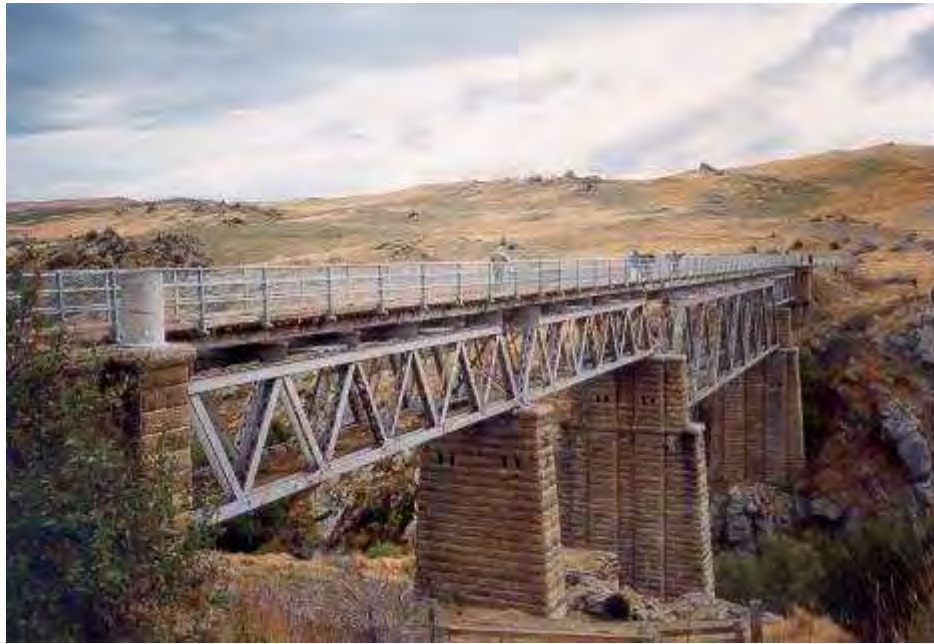
Figure 1. The impressive Poolburn Viaduct dates from 1901 and shows the detailed stone work and major engineering involved.
