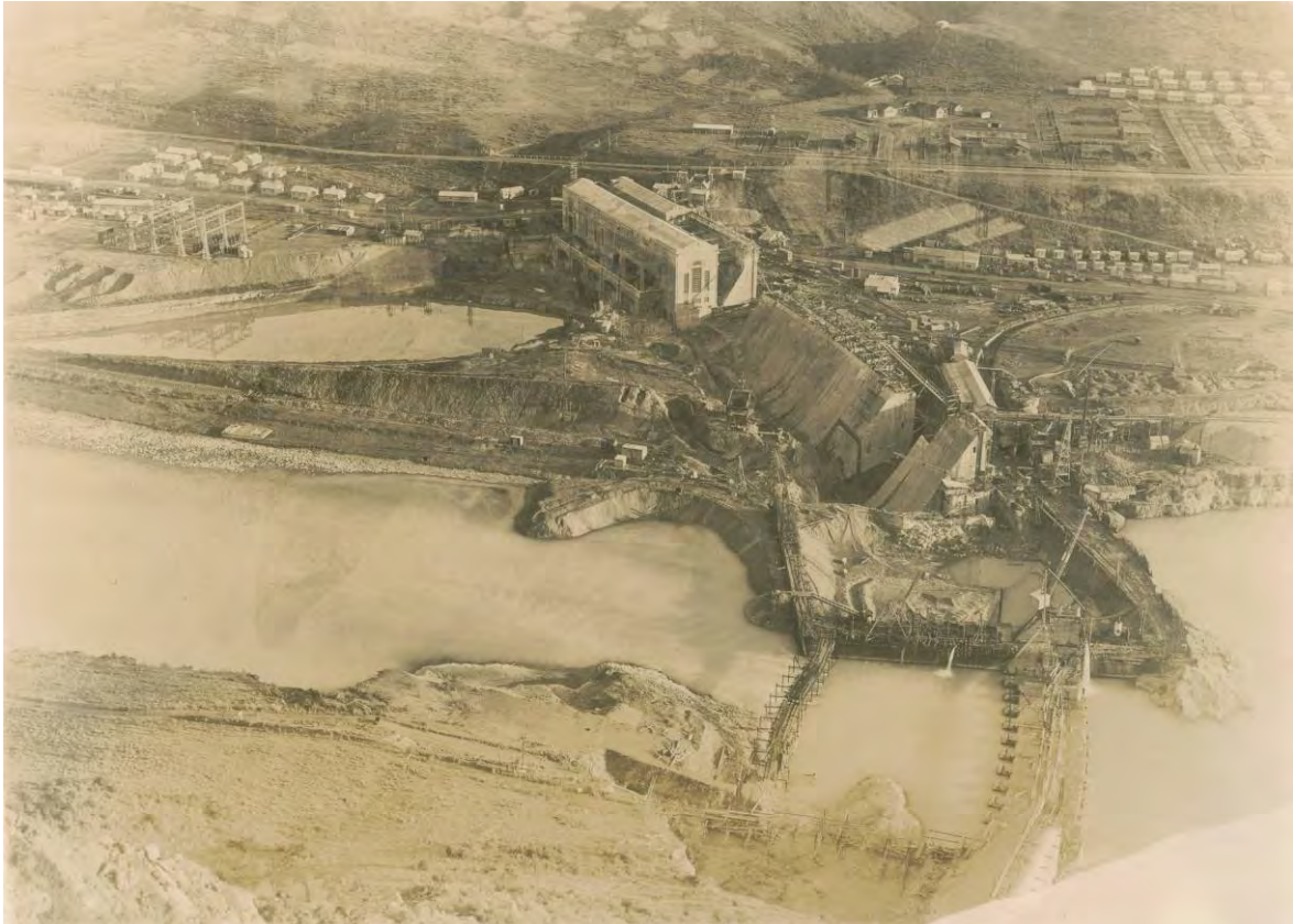
Figure 20. Initial dam blocks well advanced.
