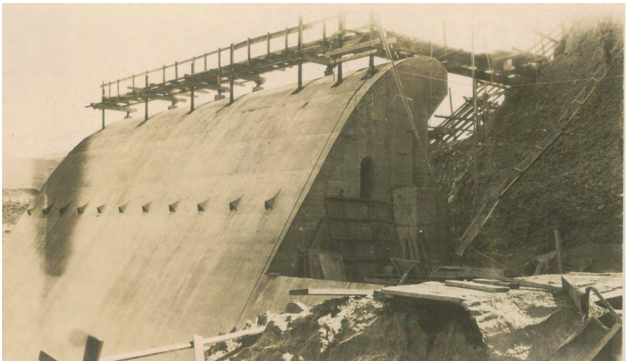
Figure 13. Left abutment block 21 showing ogee parabolic crest, air gallery and aeration ports. Excavation through surficial gravel to expose rock foundation also shown in this view.
