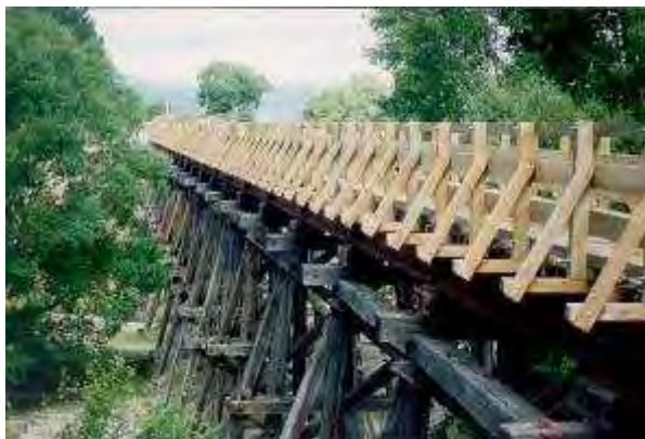
Figure 12. Muttontown Viaduct near Clyde showing raker bracing.
