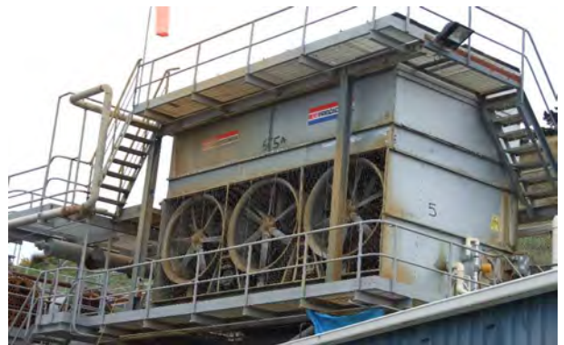
Figure 12: An evaporative condenser in service at a meat freezing plant.
