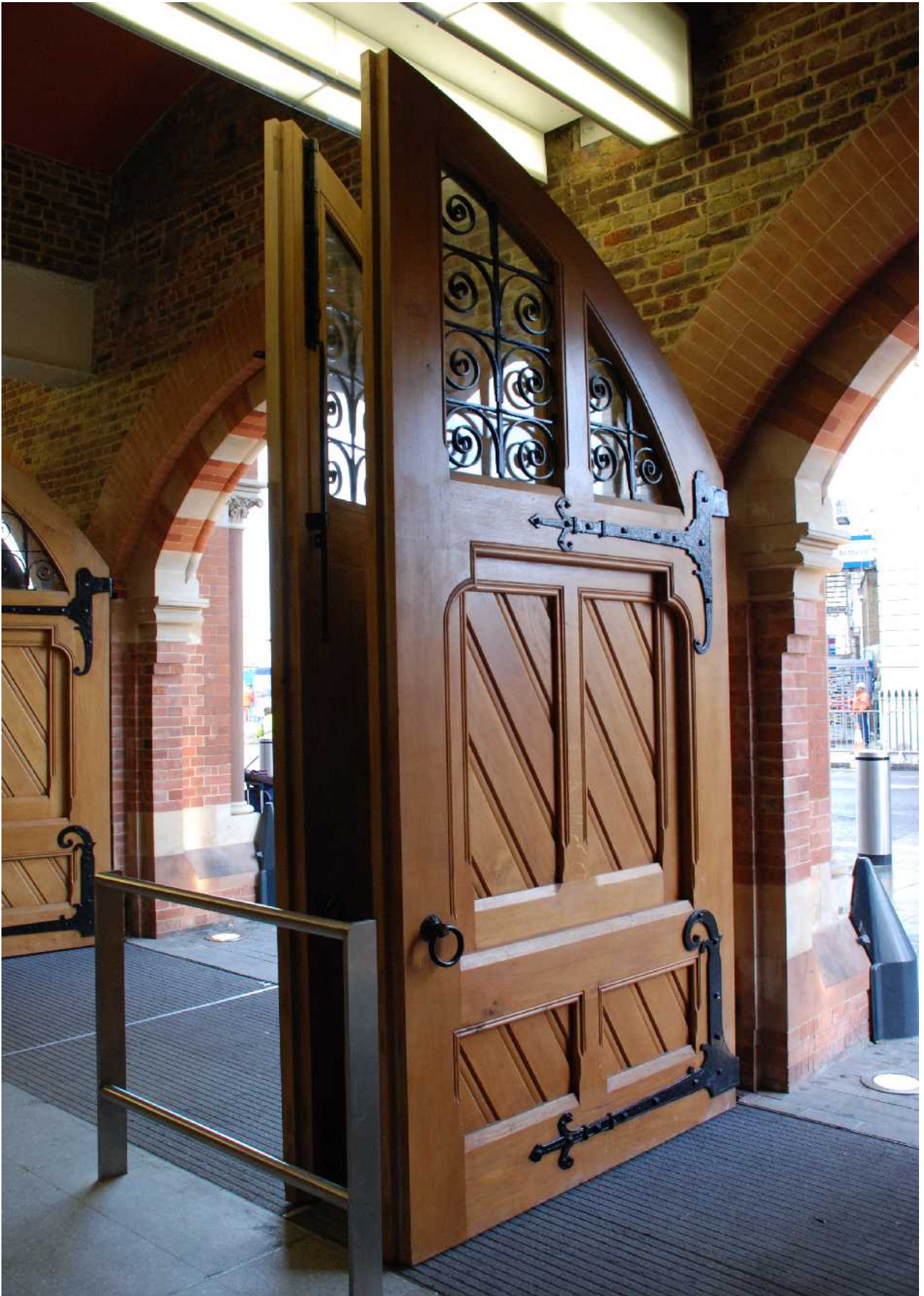
Replacement doors and other detailing at St Pancras follows faithfully William Barlow's original designs and materials.
