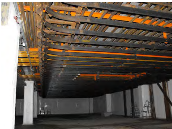
Figure 1: Carcass freezing room reliant on natural convection heat transfer to bare pipe evaporator overhead.
