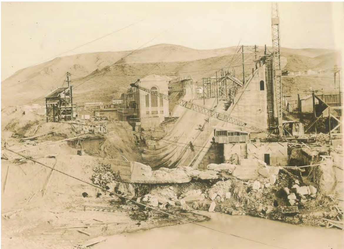
Figure 21. Closer view of initial Otago Blocks and substantially completed Power House structure in background. River bank armouring in foreground about to be removed.
