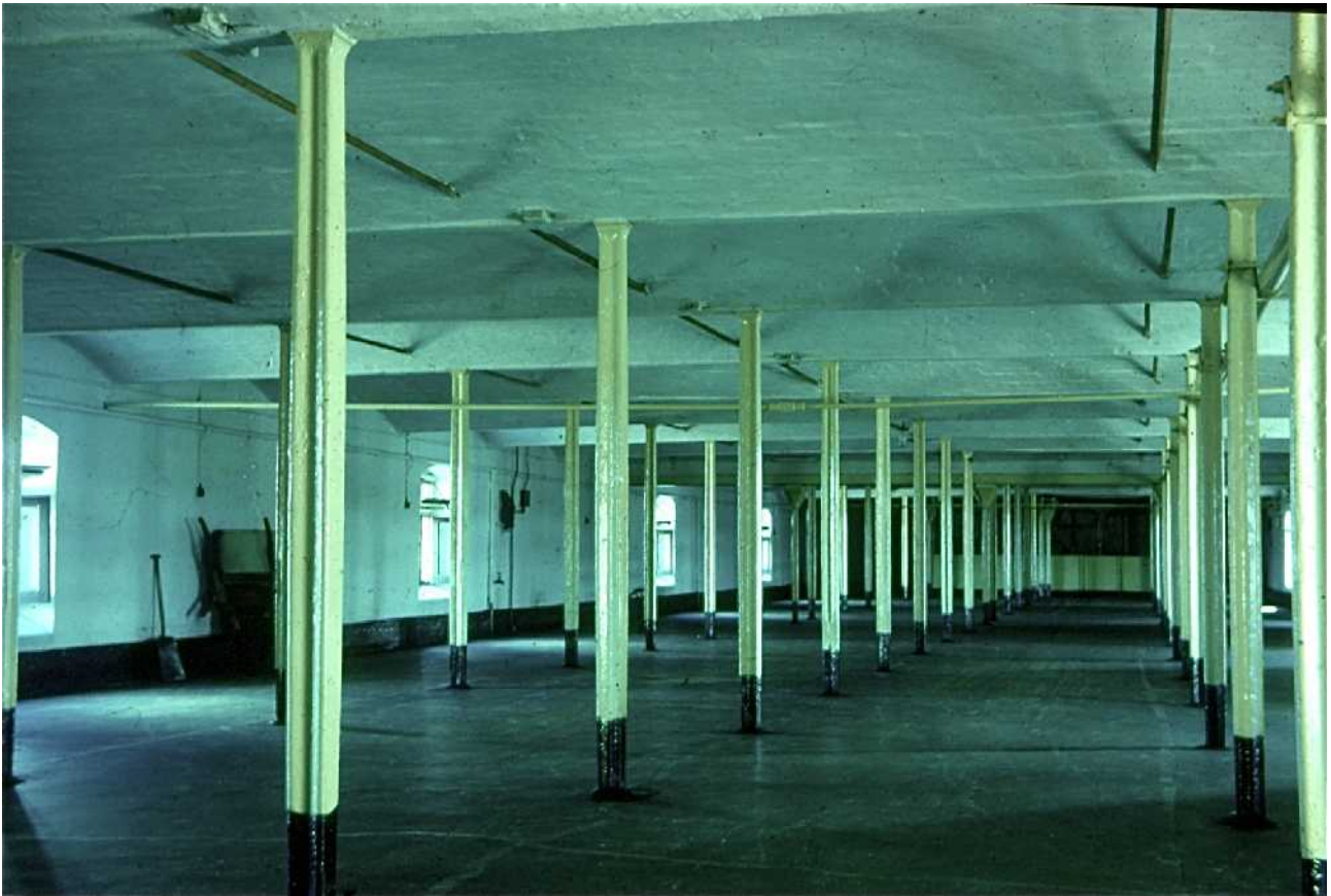
Ditherington Flax Mill, Shrewsbury, the world's first iron-framed building (1796/7). Out of use for nearly thirty years the mill is undergoing structural repairs by English Heritage prior to a new use being found.
