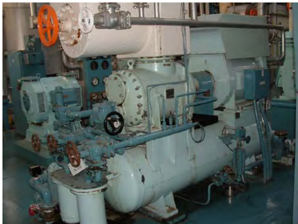
Figure 10: A relatively early model twin screw compressor
