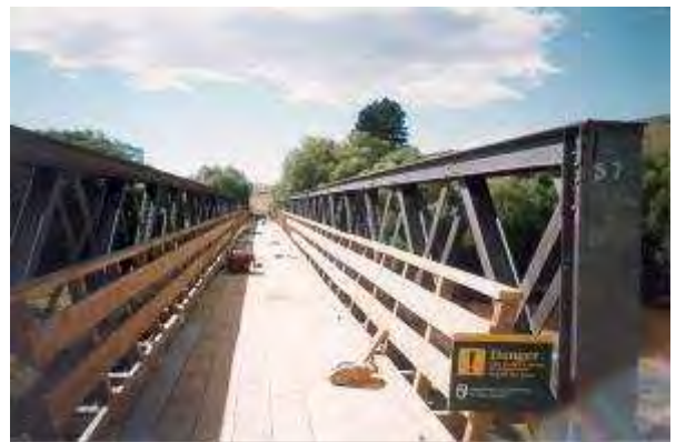
Figure 9. Waipiata Bridge being re-decked for cyclists and walkers.
