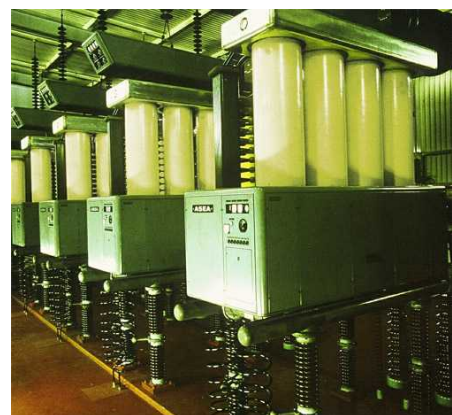
Figure 6 Mercury-arc valves
