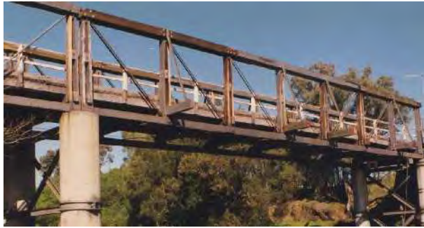
De Burgh (Pratt) composite truss bridge
