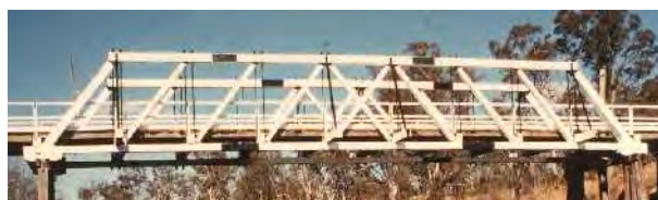
Timber Howe truss
