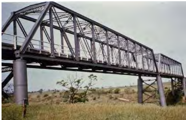
Figure 8. The 1905 steel Pratt trusses for the Luskintyre road bridge over the Hunter River near Lochinvar. Note
