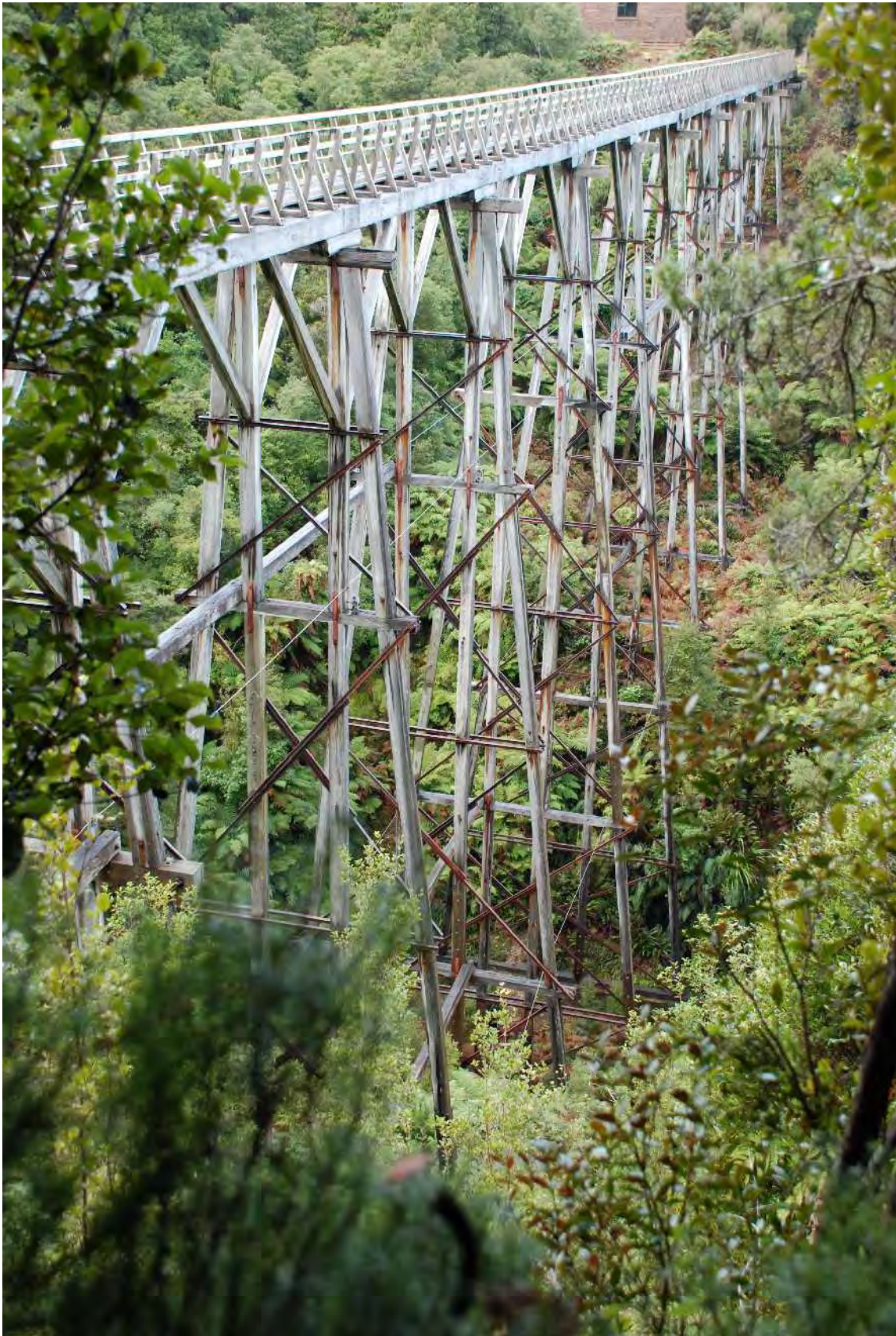
Timber viaducts, once common as first generation railway bridges in North America and Australasia, are now extremely rare. This example, Percy Burn Viaduct, behind Port Craig, New Zealand is recognised by IPENZ for its heritage value.
