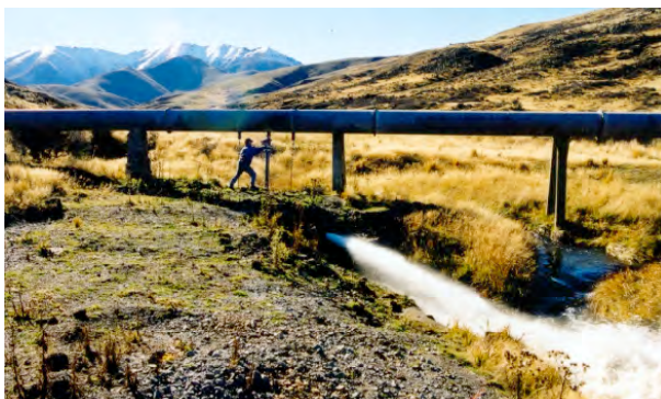
Figure 7. Wetherburn syphon sluice valve in operation
