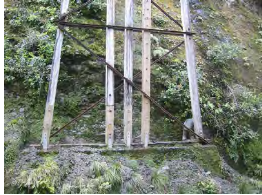
Figure 6. Previously repaired pier columns with laminated spliced timber
