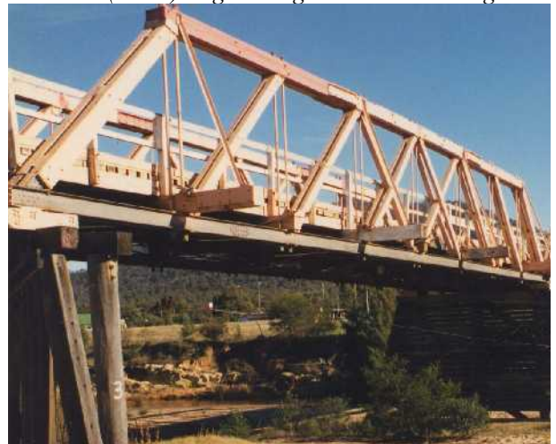
Dare (Howe) composite truss bridge [Fig.7 continues]
