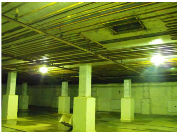
Figure 2: Cold store cooled by overhead bare pipe evaporator.
