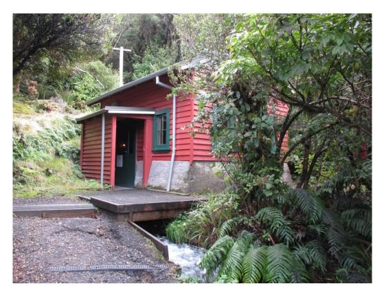
Path providing access to the power house. A push button light illuminates the interior so the public can see the machinery in action. The tailrace is in the foreground. Natasha Naus, 2015.
