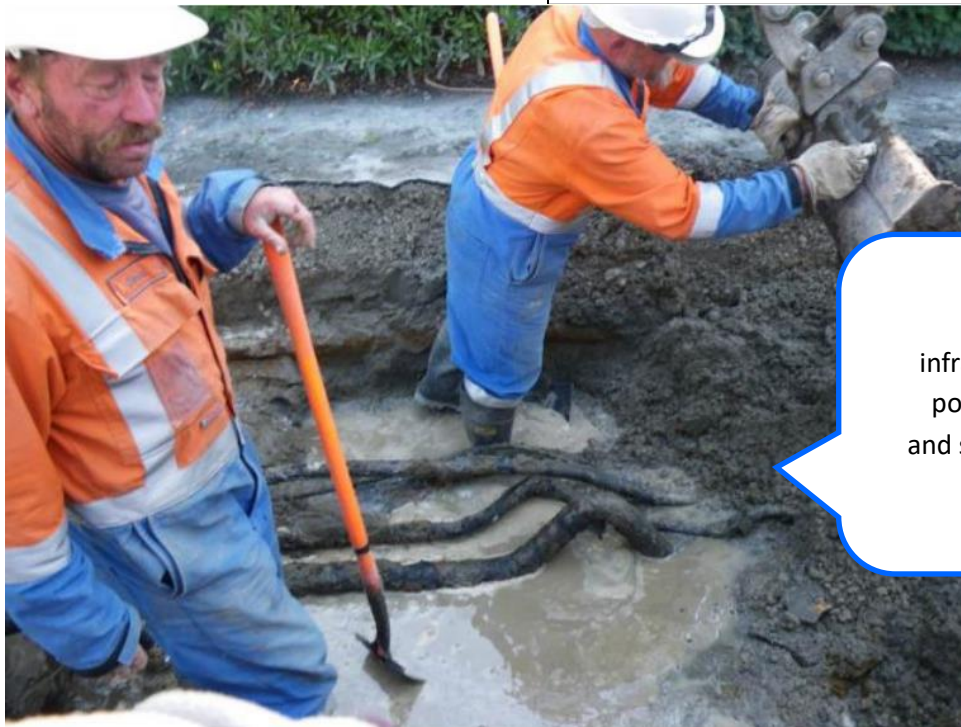
Figure 6: Earthquake damaged 11 kV steel and lead armoured cable, and above embedded in fractured concrete, a damaged 66 kV oil-filled cable.
