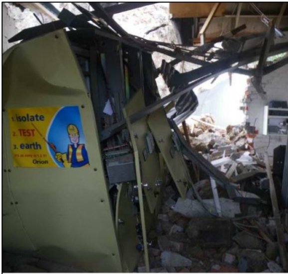
Figure 4: Sumner substation boulder damage.
