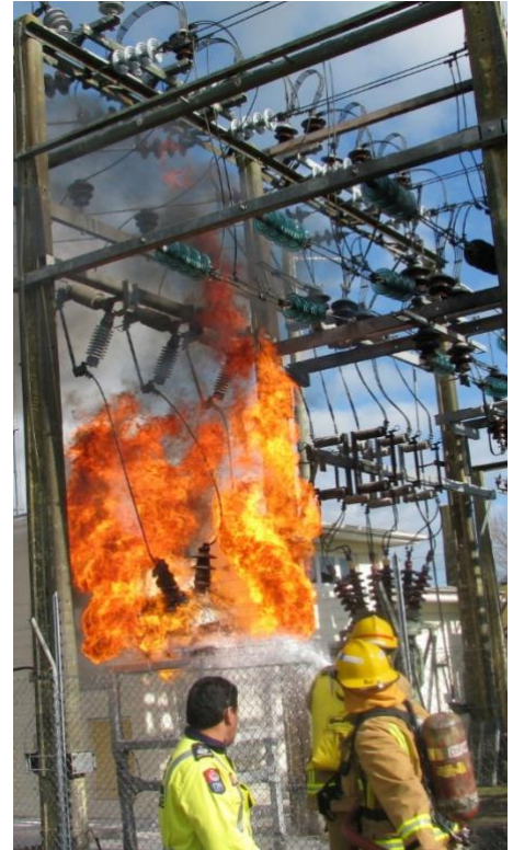
Substation fire. Source: Bruce Mills
